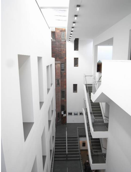
Fig 2. Atrium added in 2005
