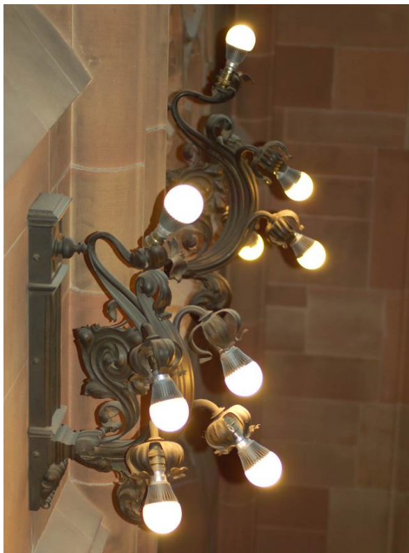
Fig 29. Original light fitting
