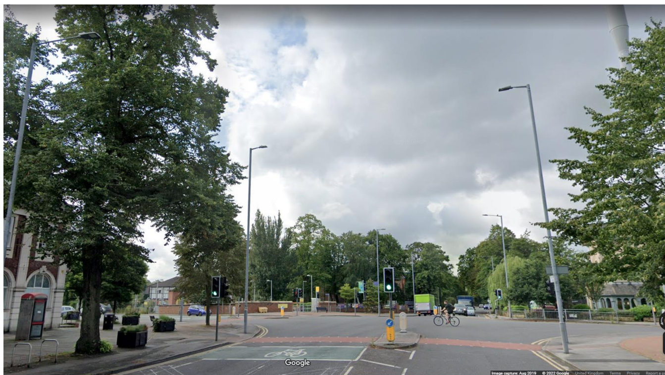
Looking at the site from Palatine Road on the north-east of the site towards the west and Pipe Bridge. (Source: Google)
