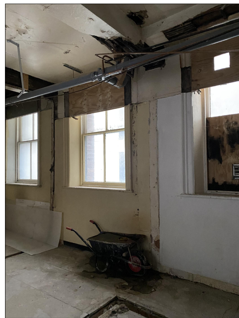
IMAGE 1 Existing lath and plaster repairs to holes in beam encasement and adjacent ceilings. New MF plasterboard underdrawn to these areas
