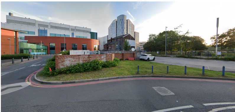
View from North Road toward the existing Car Park
