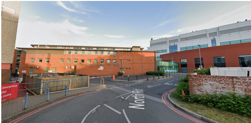
View from North Road toward the Wellcome Centre
