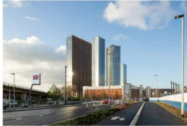
View of the Premier Inn Hotel currently on site, taken from the Mancunian Way - click to enlarge
