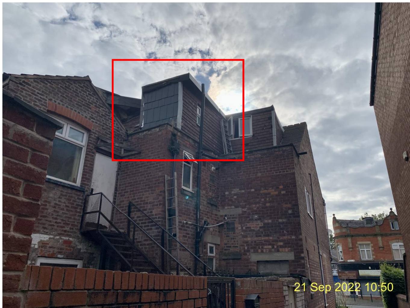
Photograph 3 Shower room as observed from the side alleyway between 267 Moseley Road and Moseley Court
