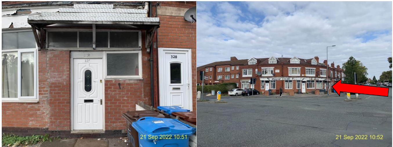
Photograph 2 Front Entrance to 330 Slade Lane. Source Case Officer Photographs date as shown.
