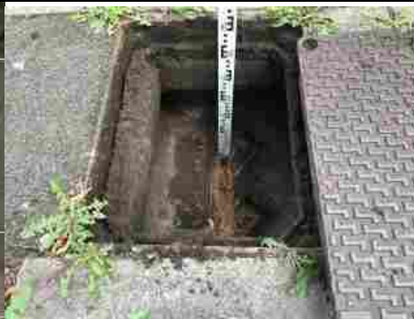
Photograph 13 A 0.72m deep manhole by the building entrance.
