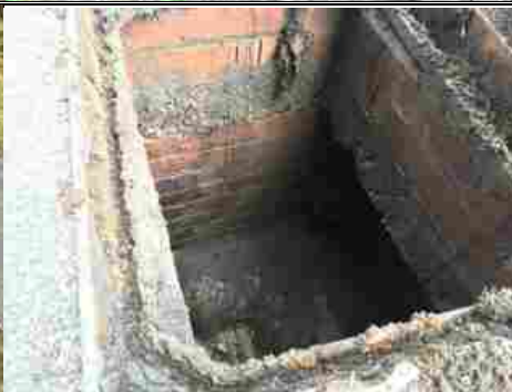
Photograph 14 A 1.3m manhole further towards York Avenue, with a site drainage outfall.
