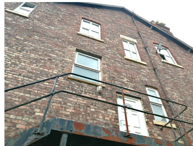
Brickwork to be repaired, cleaned and repointed.
