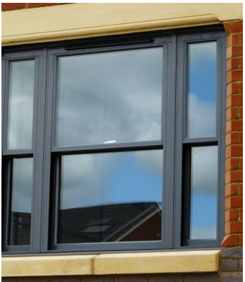
Slim line Aluminium vertical sliding slash window
