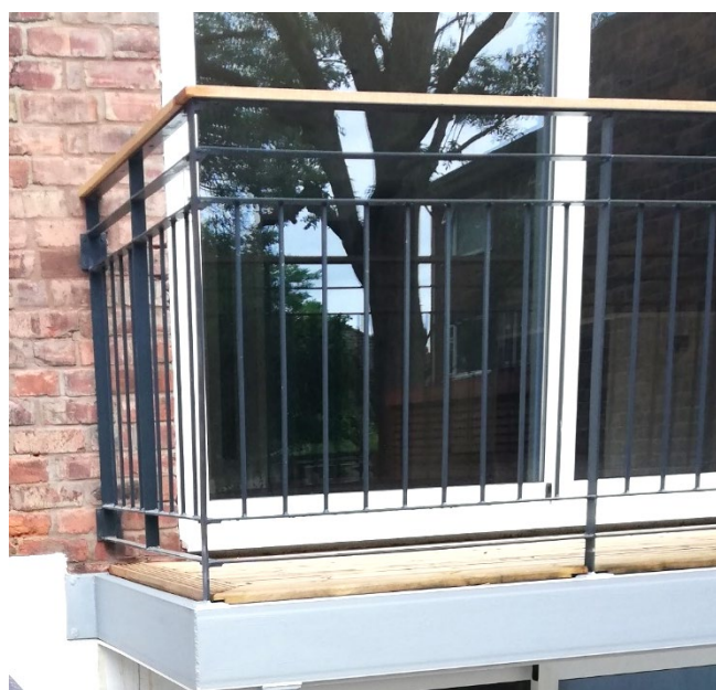
Metal balustrade to balconies galvanised and painted dark grey with Oak hand rail capping.
