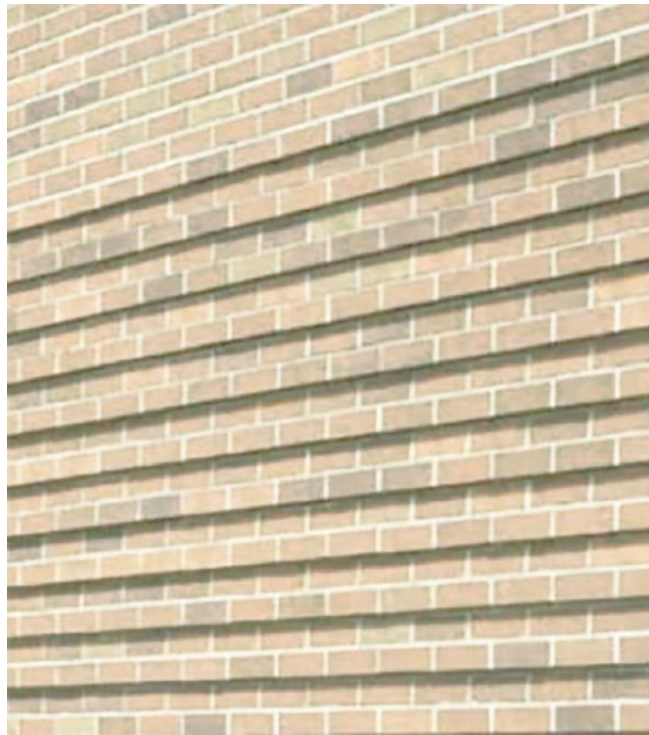
Brickwork Texture detail
