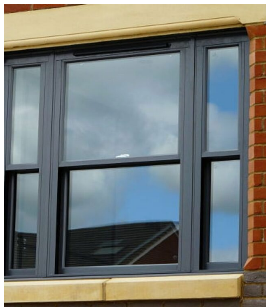
B: Slim line Anthracite Aluminium vertical sliding slash window
