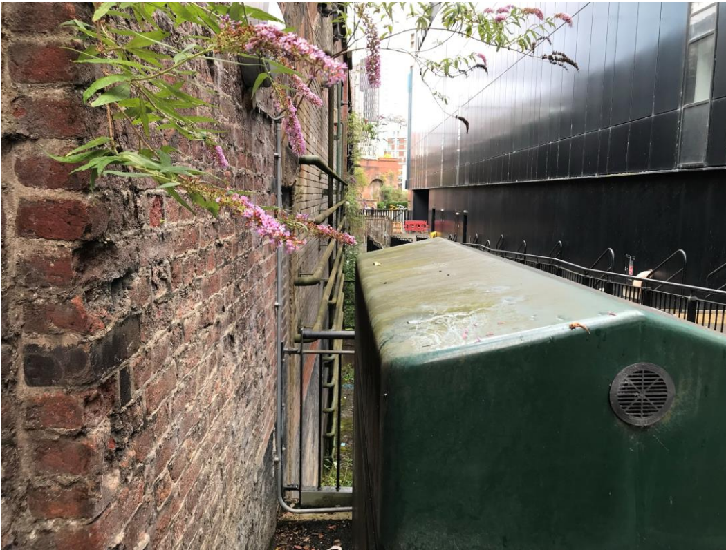
30) Overview of the rear infill with the neighbouring retaining structure in close proximity.
