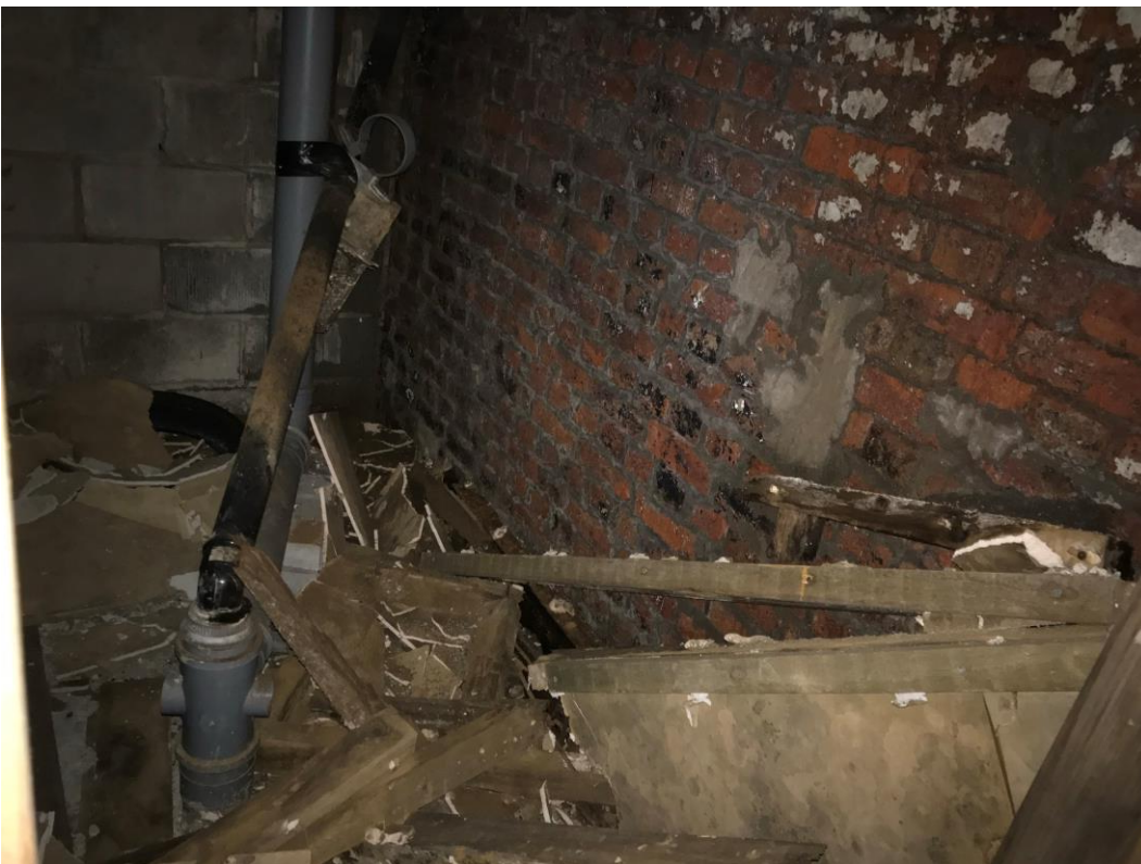
22) Debris to basement level. Location of existing foul waste which will be connected into as part of the WC construction works.
