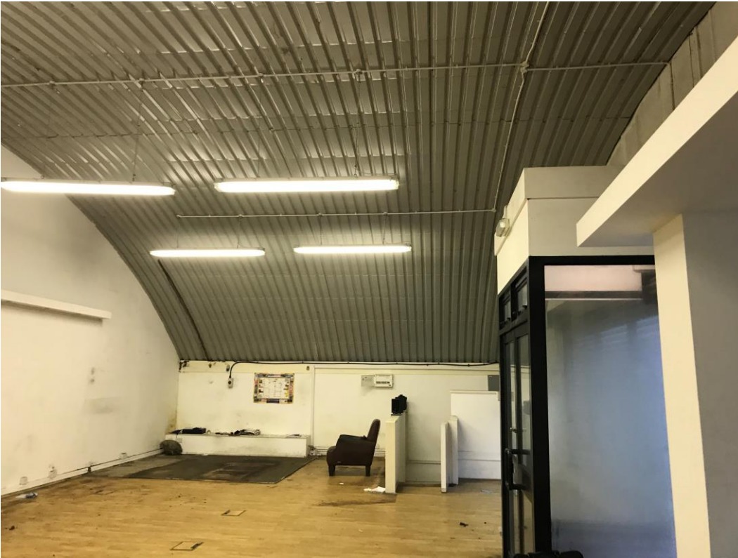
13) Overview of shop floor which has been formed from the existing mezzanine structure.
