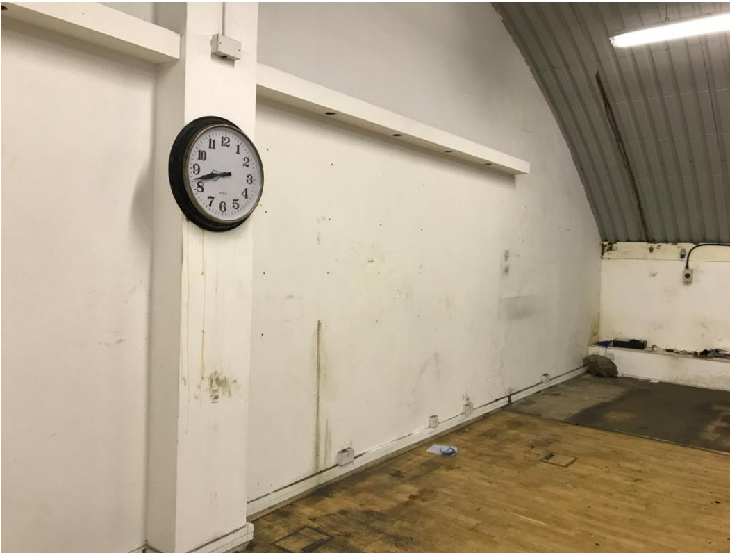
19) Overview of shop floor which has been formed from the existing mezzanine structure.
