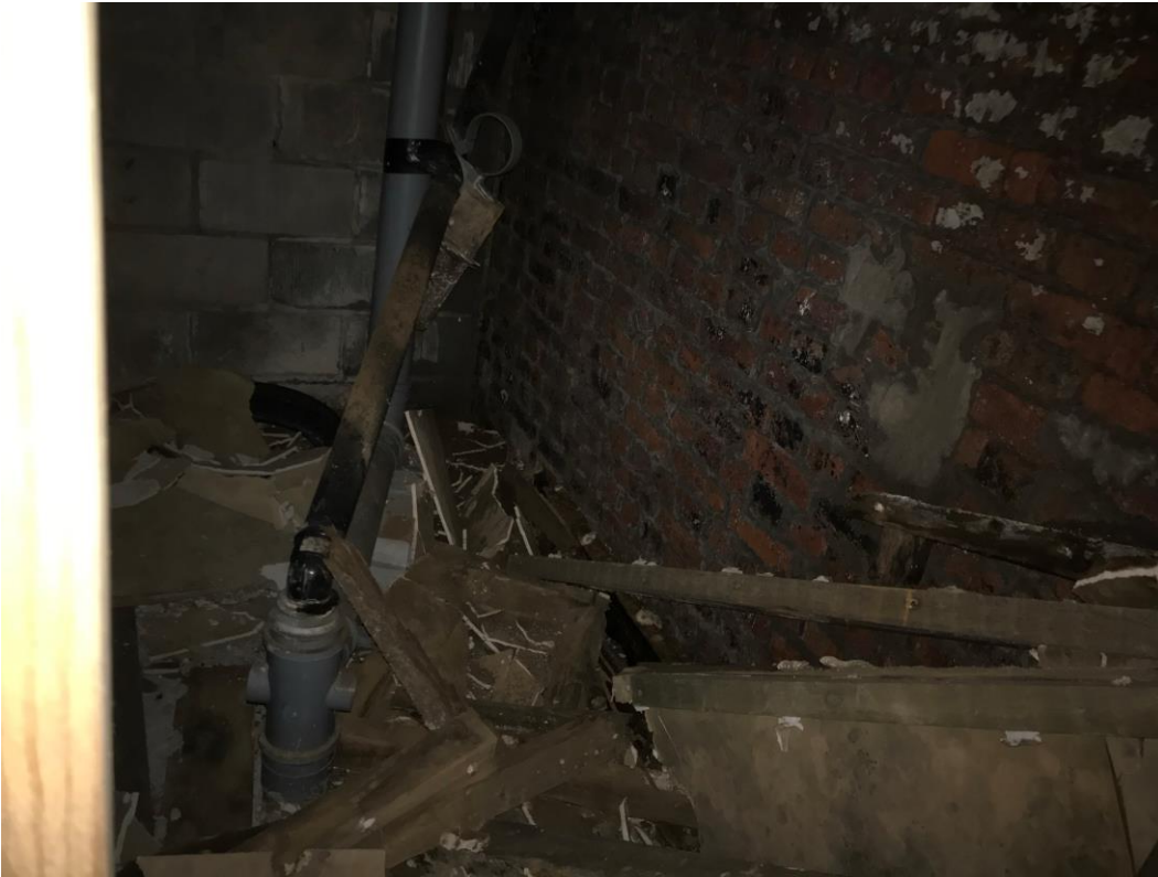
21) Debris to basement level. Location of existing foul waste which will be connected into as part of the WC construction works.
