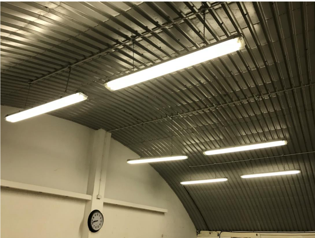
14) Overview of ceiling lining and lighting system.
