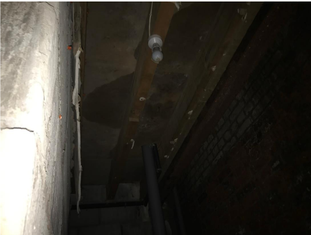
24) Underside of the mezzanine structure, which is damp affected and not fit for purpose.
