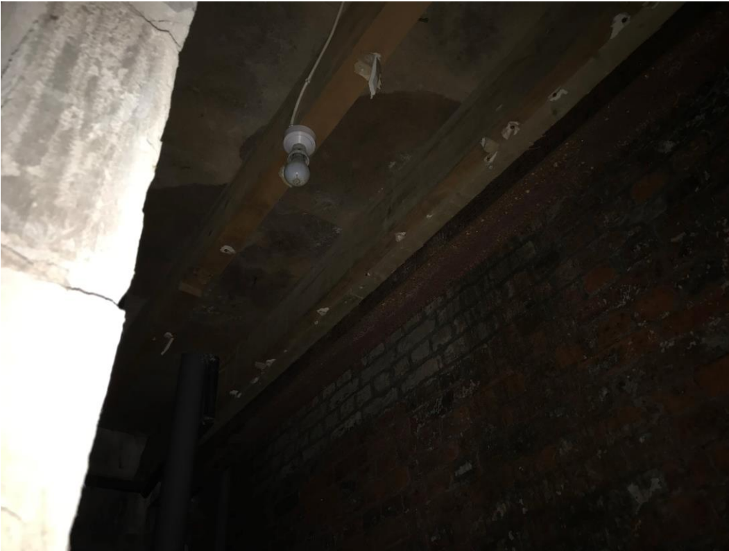
26) Underside of the mezzanine structure, which is damp affected and not fit for purpose.
