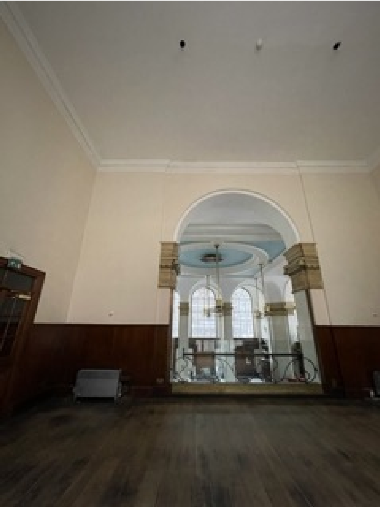
06 SITE PHOTO - FREE STANDING UNIT NEXT TO HERITAGE PANELLING DE-08 Scale: Actual Size
