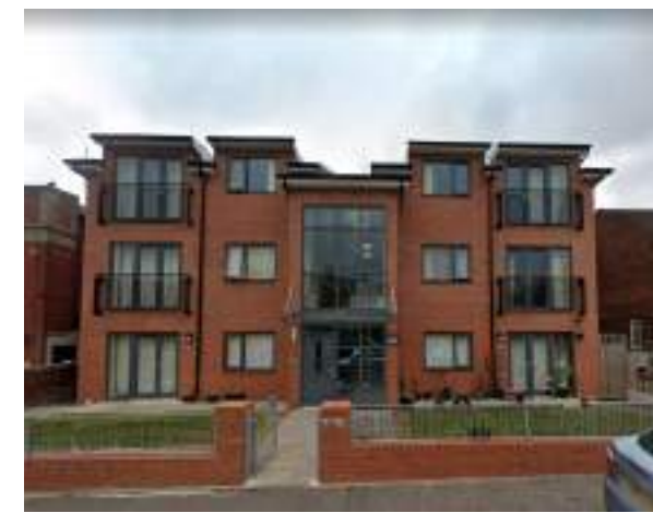
5 - Green Street - 3 storeys
