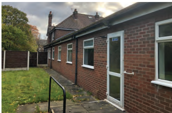
Photo: Existing East-Facing Windows
