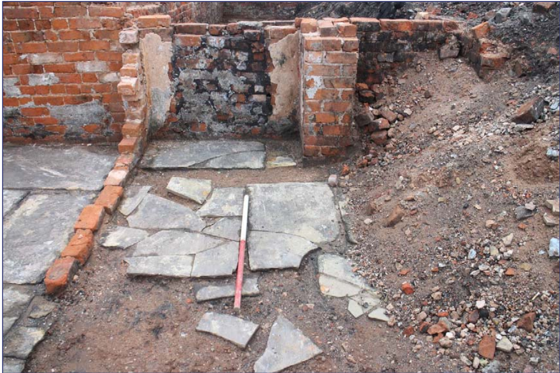
Plate 24: Southern elevation of C4 , with patches of surviving lime plaster
