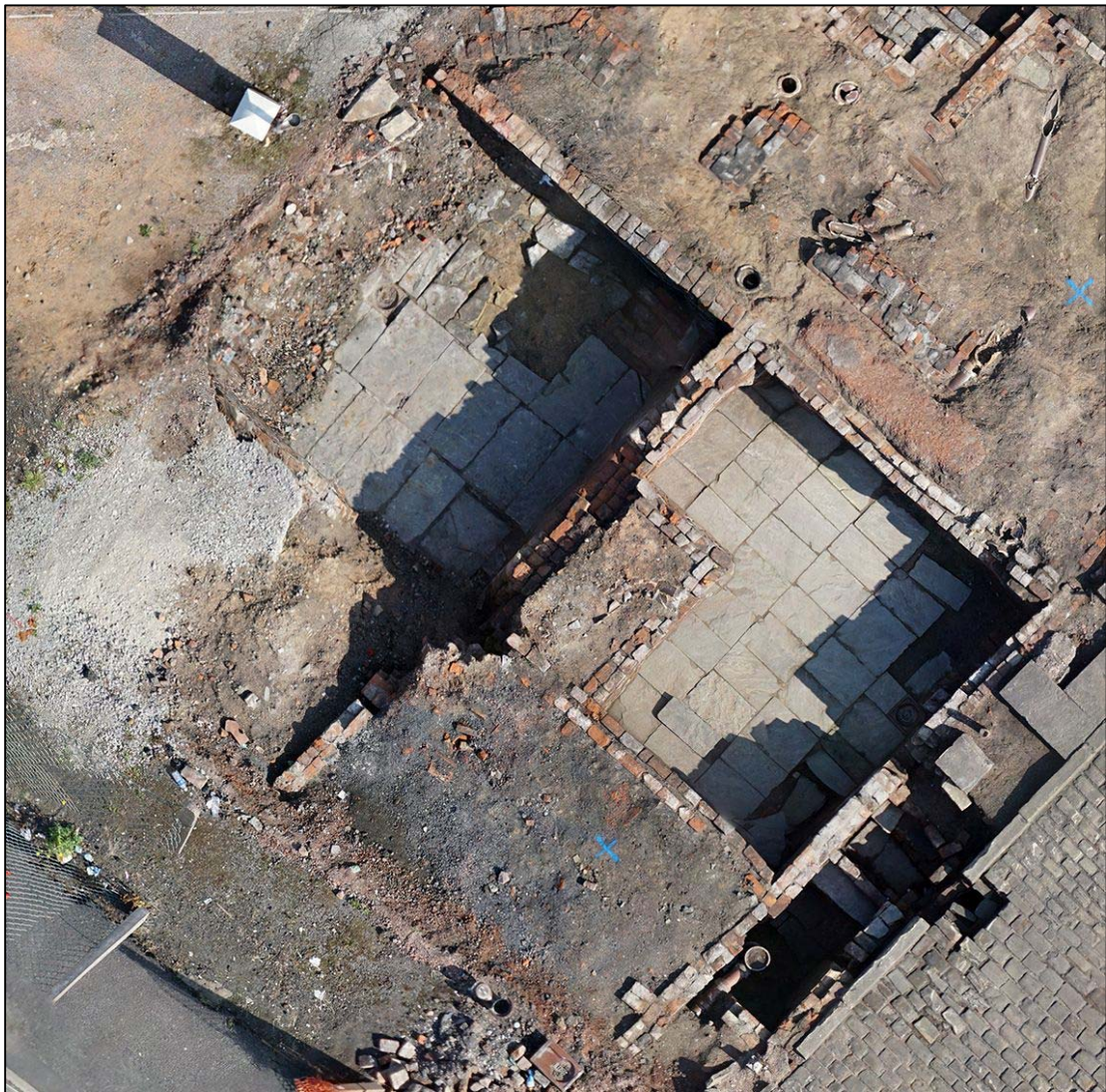
Plate 49: Aerial view of C1-3
