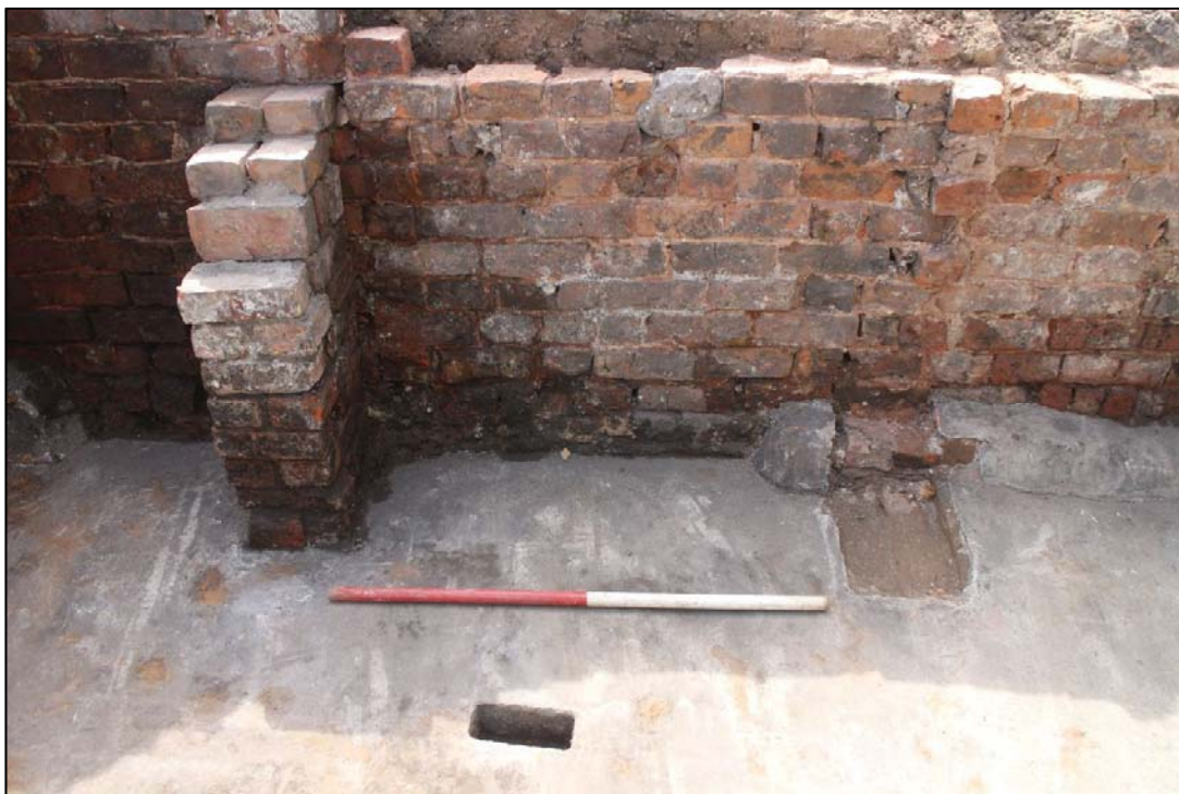
Plate 69: Remains of the fireplace in C1, looking south-west
