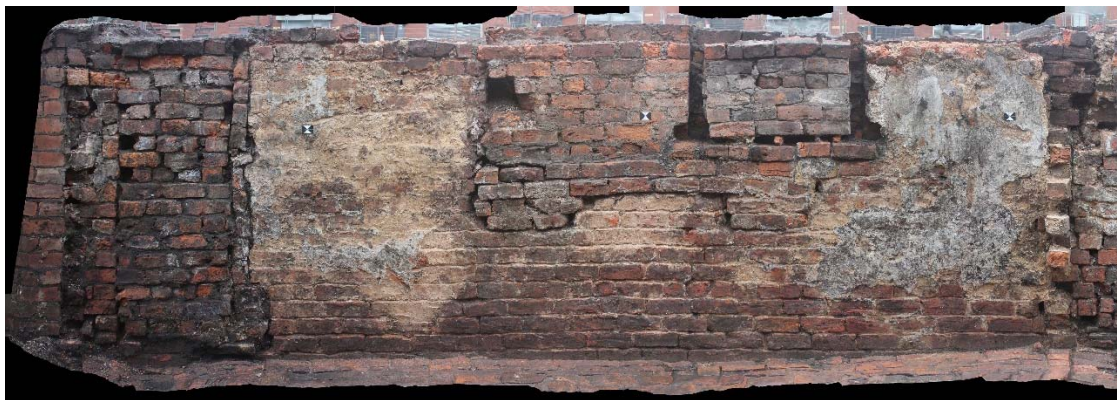
Plate 74: The north-west-facing elevation of C4 , showing the Phase 1 wall and door, and the Phase 3 cellar light (later blocked)
