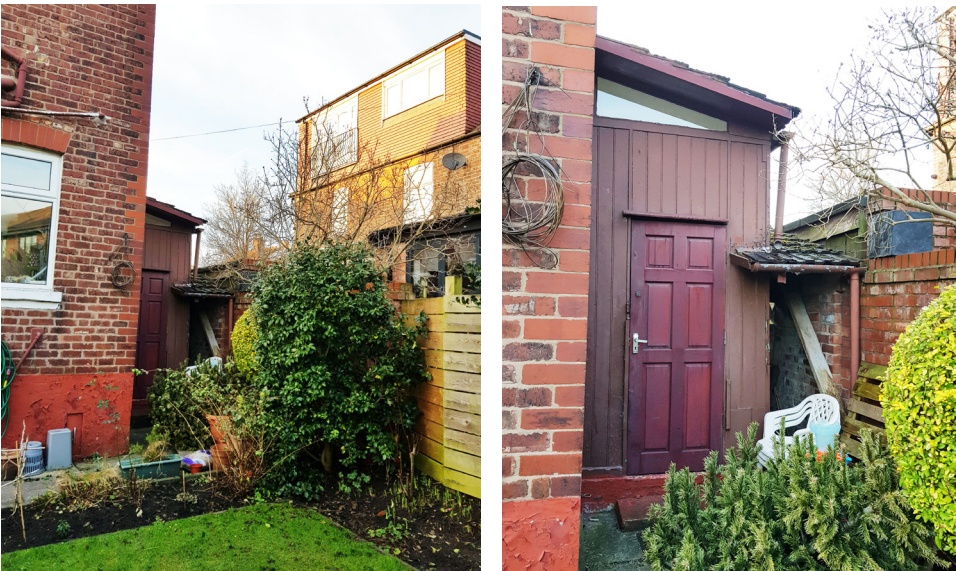
Existing Northern neighbouring wall and close up view from rear
