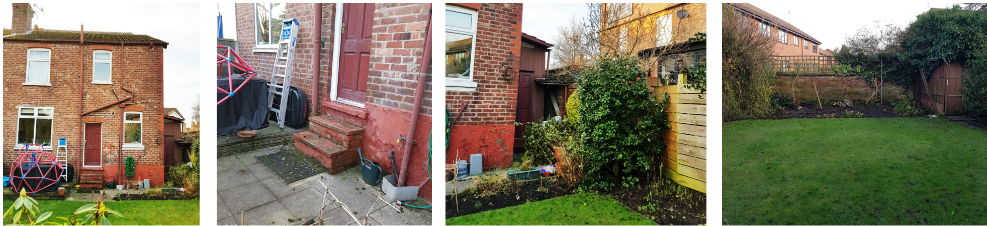
Existing building photos
