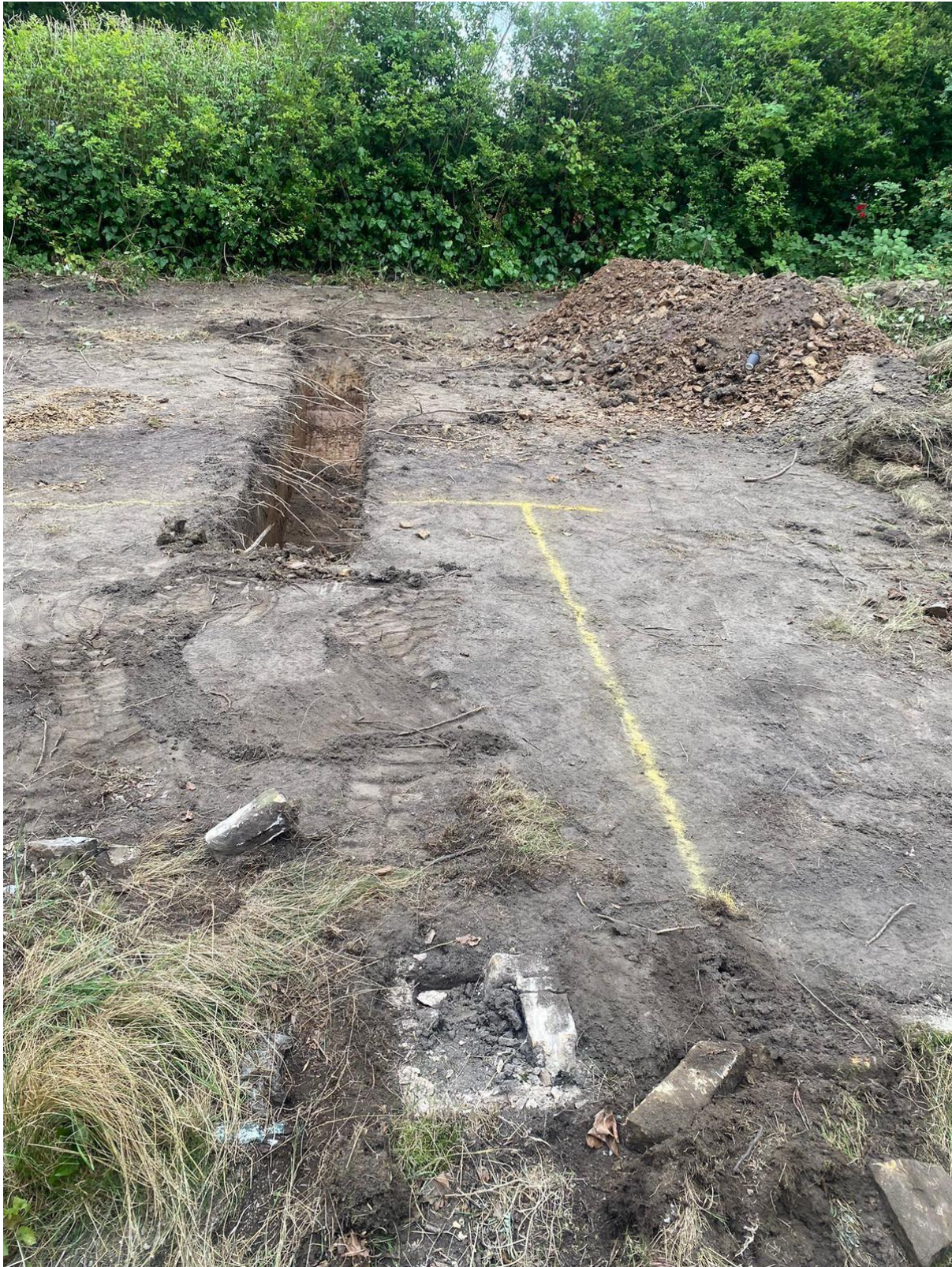
Above is a photograph showing the excavation for the foundations of Plot No. 4.
