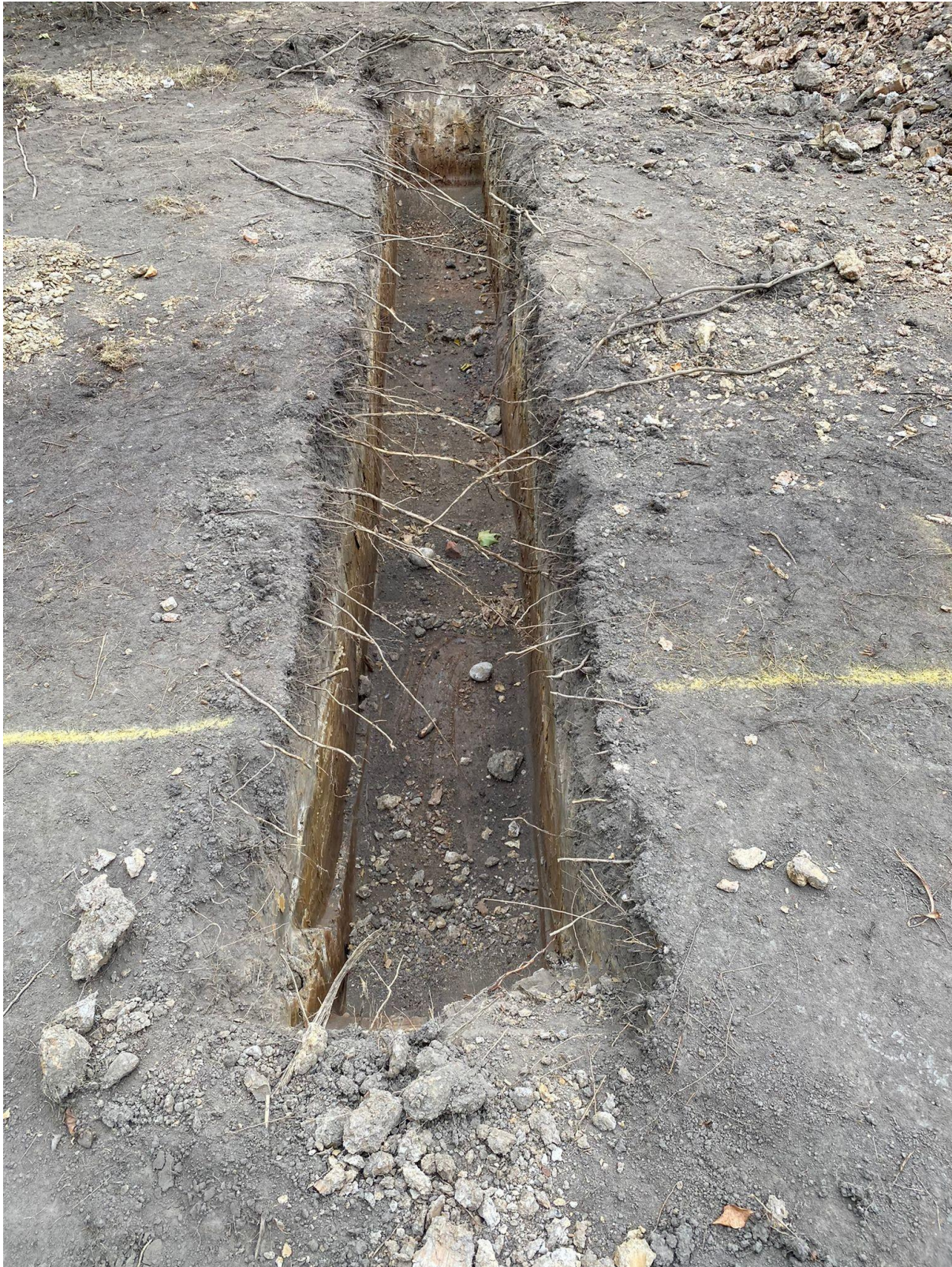
Above is a view looking at the foundation footings following excavation works.
