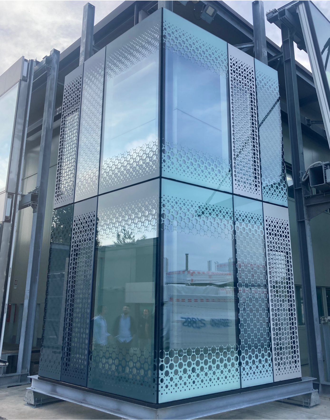
VISUAL MOCK UP - BUILDING D Photographed 12.10.2022
