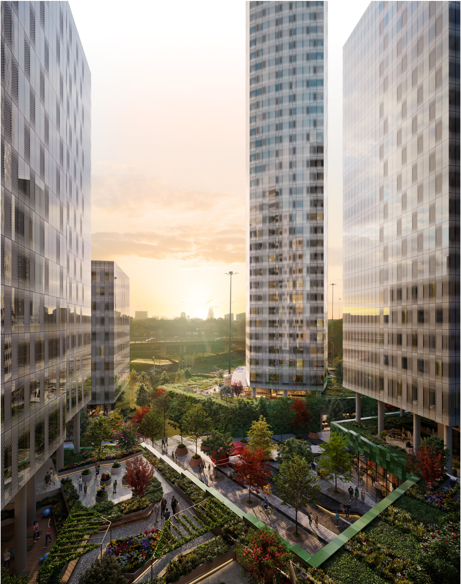
View from Building B looking across the landscape podium towards Mancunian Way
