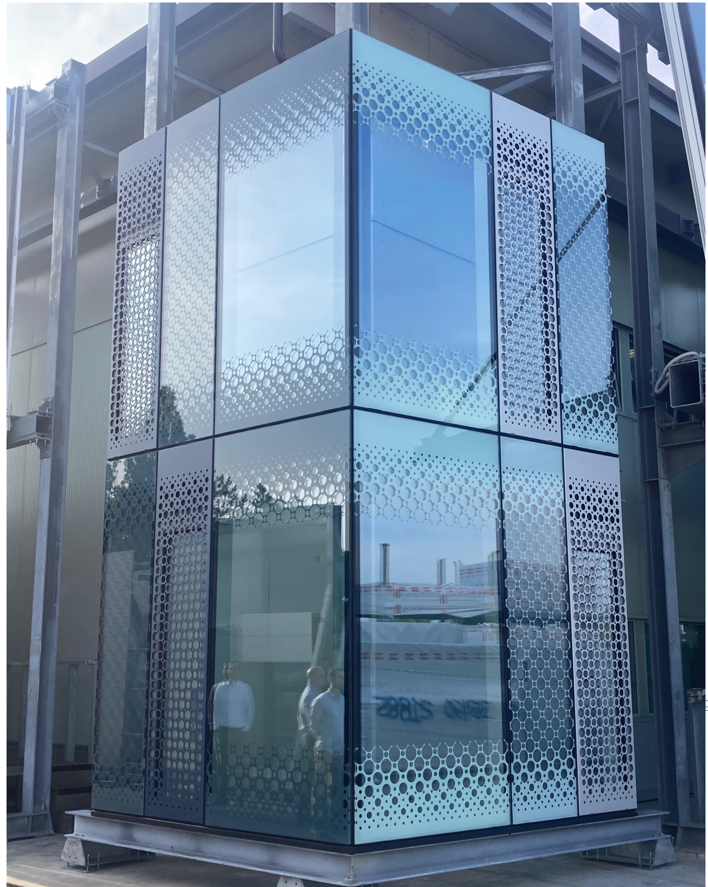
VISUAL MOCK UP - BUILDING D Photographed 12.10.2022
