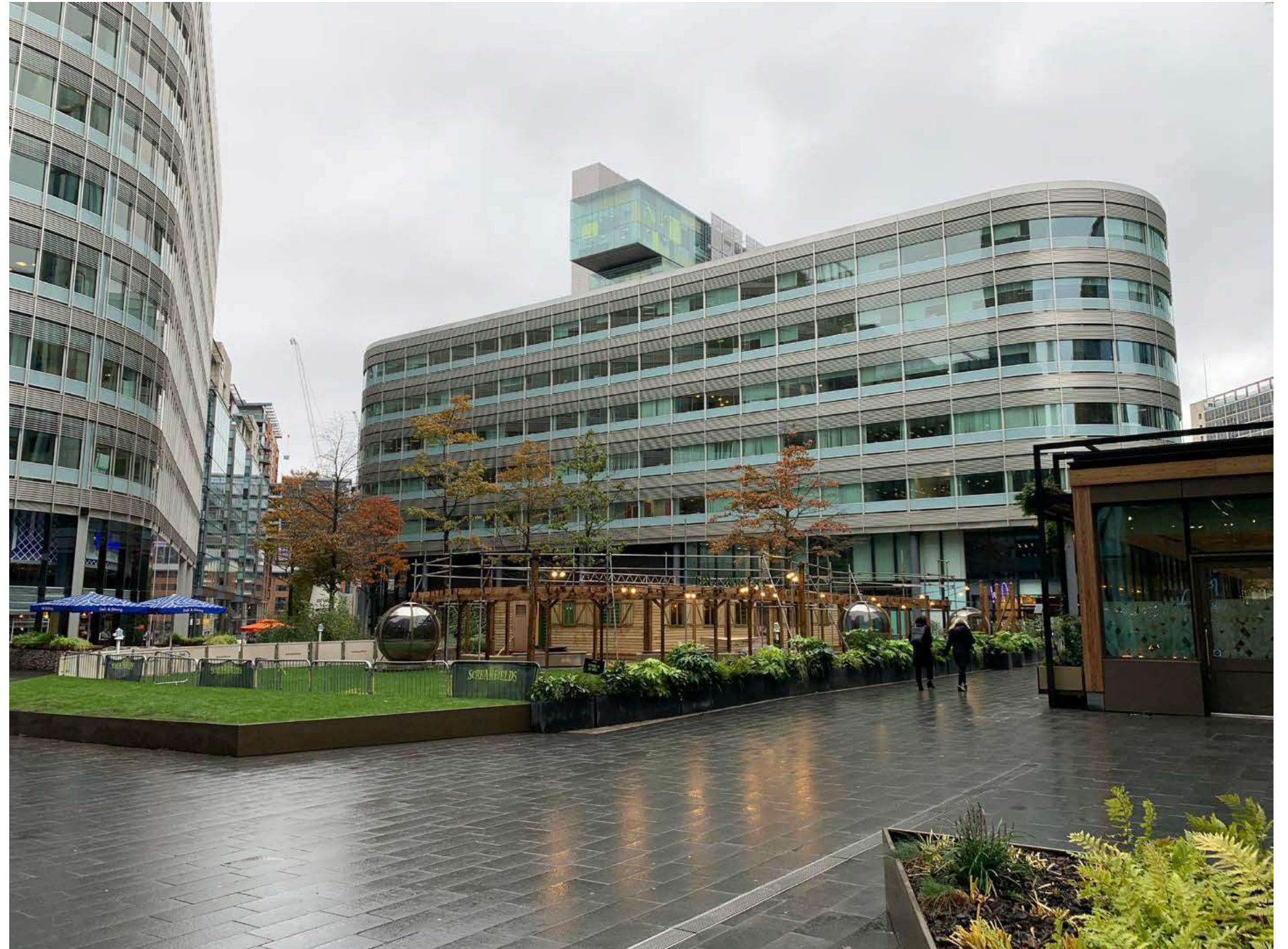
Figure 1. External photograph of 4 Hardman Square (as existing)
