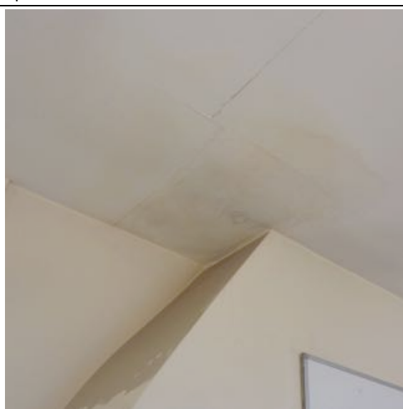
Stain to the ceiling the west of the chimney stack. This is currently dry though
