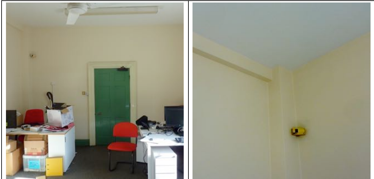
General view looking East. In the left corner is a nib and a beam along the ceiling. This may date from when this was open plan and used as a shop?
