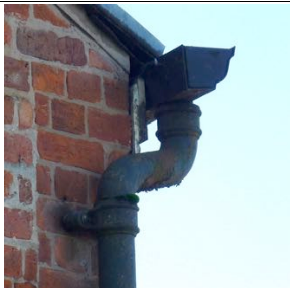
View of the downpipe which has to take all of the water from the south and west roof pitches. The rust would suggest this is often blocked and overflowing.
