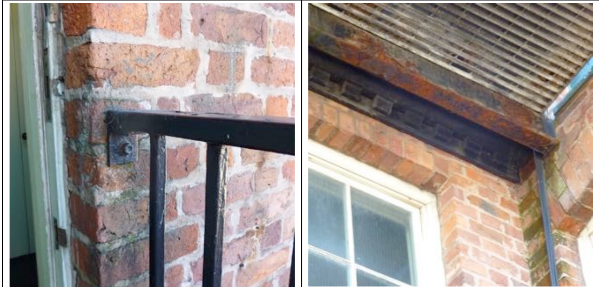
Ferrous fixings for the end of the access bridge to the gable wall. Bolts are into the joint not the brick.
