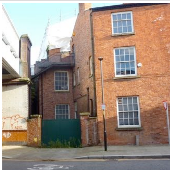
The damp staining to the boundary wall at low level may be where the over-topping rainwater pipe drops its water.
