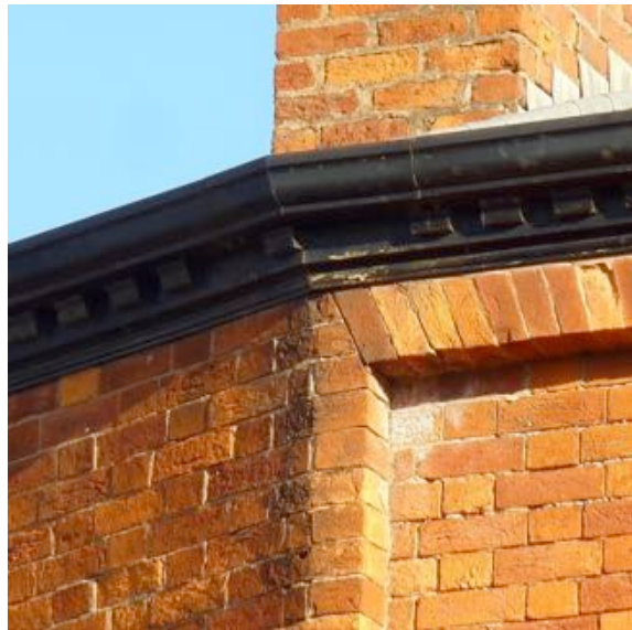
View up the corner of one of the faceted sections. This looks to be quite precise with no distortion.
