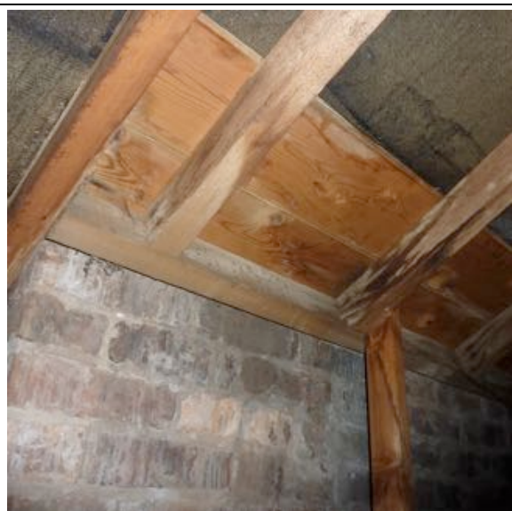
North wall evidence of past leaks around back gutter of chimney stack. Currently all dry.
