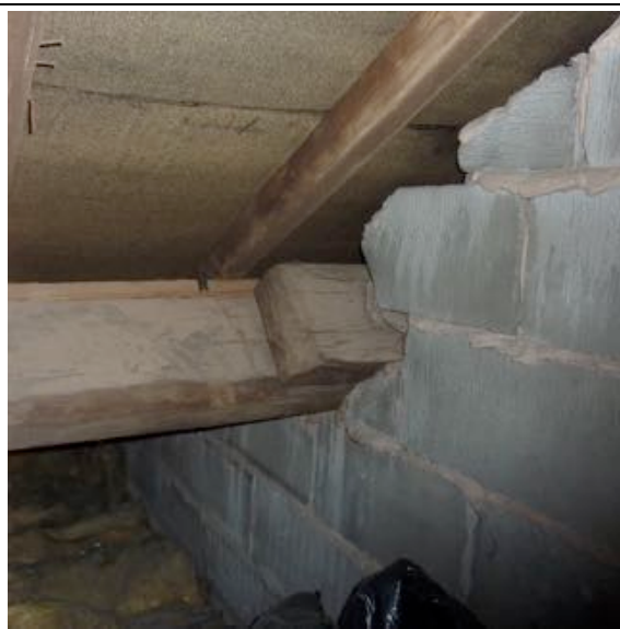
General view looking west to blockwork partitions. South purlins supported by blockwork wall, would this once have been a timber truss?
