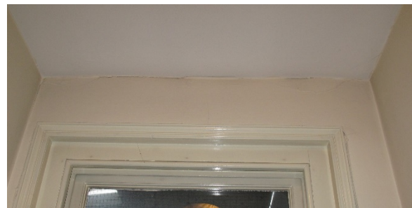
FIRST FLOOR REAR WINDOW OPENING
