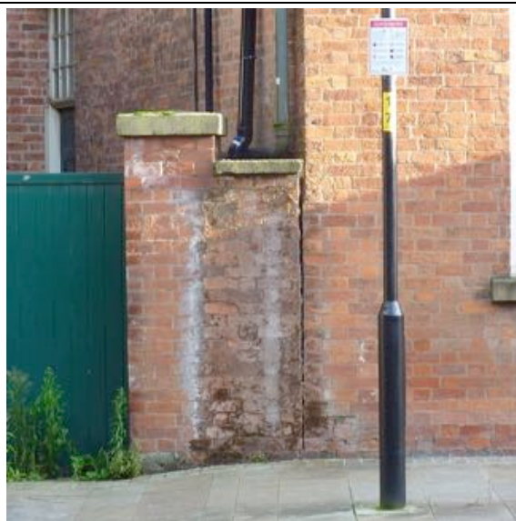
The damp staining to the boundary wall at low level may be where the over-topping rainwater pipe drops its water.
