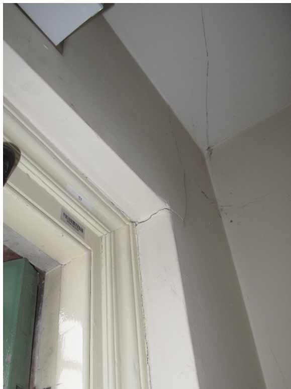
SECOND FLOOR REAR DOOR OPENING
