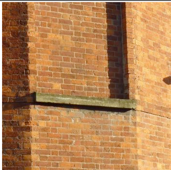
Detailed view of the brickwork to the facet areas. Widespread washing out of the mortar to the upper areas.
