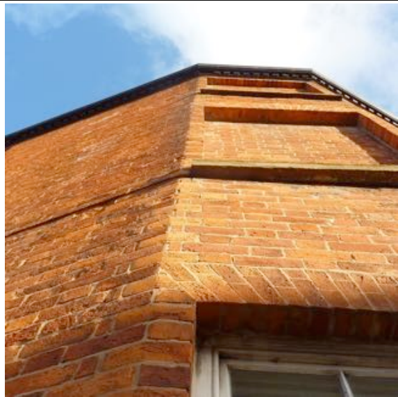
View up the corner of one of the faceted sections. This looks to be quite precise with no distortion.
