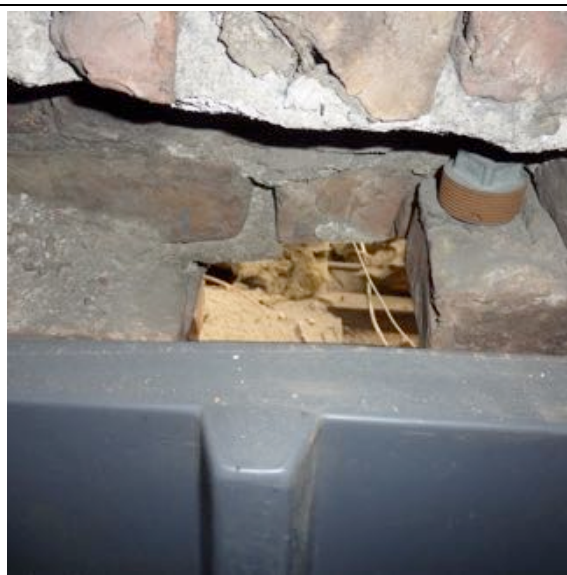
Hole in wall behind the water tank links to the adjacent station building
