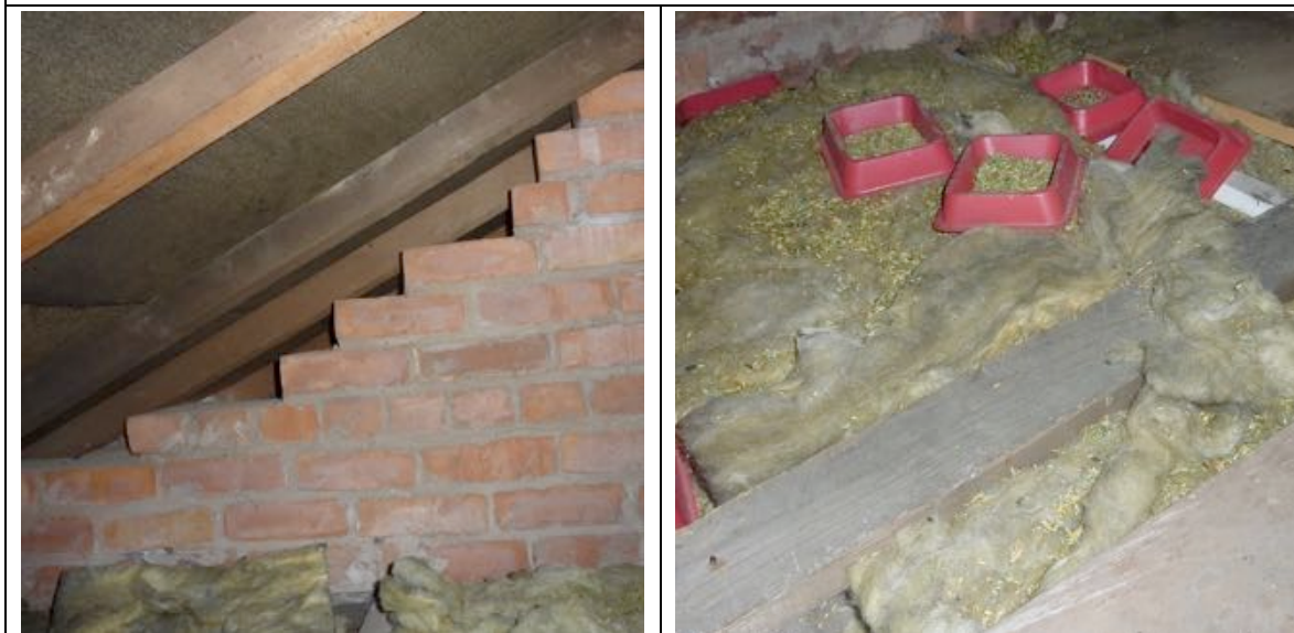
Further shots of the brickwork and plasterboard at the eaves of the faceted roof. This is all bone dry.
