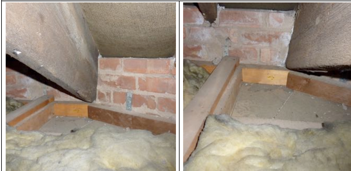
Further shots of the brickwork and plasterboard at the eaves of the faceted roof. This is all bone dry.
