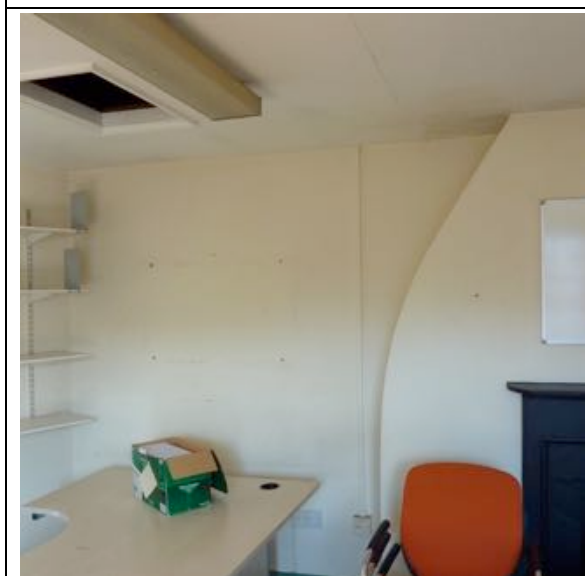
Stain to the ceiling the west of the chimney stack. This is currently dry though
