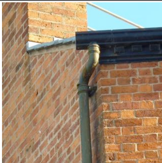
View of the downpipe which has to take all of the water from the south and west roof pitches. The rust would suggest this is often blocked and overflowing.
