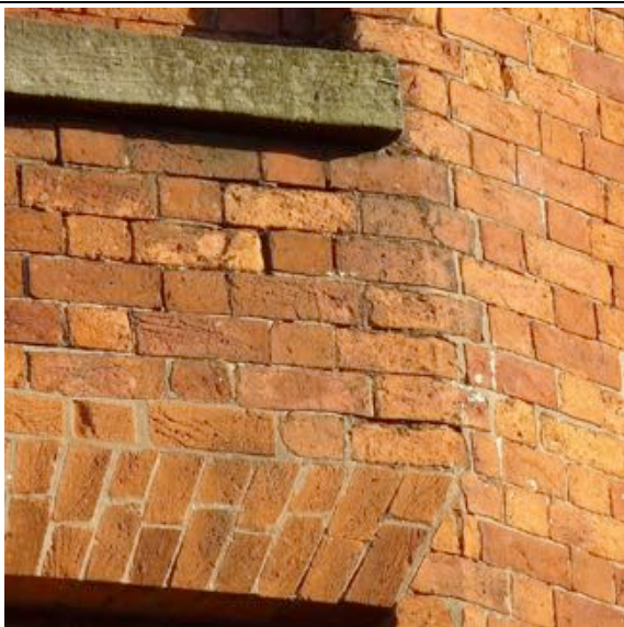
Detailed view of the brickwork to the facet areas. Widespread washing out of the mortar to the upper areas.
