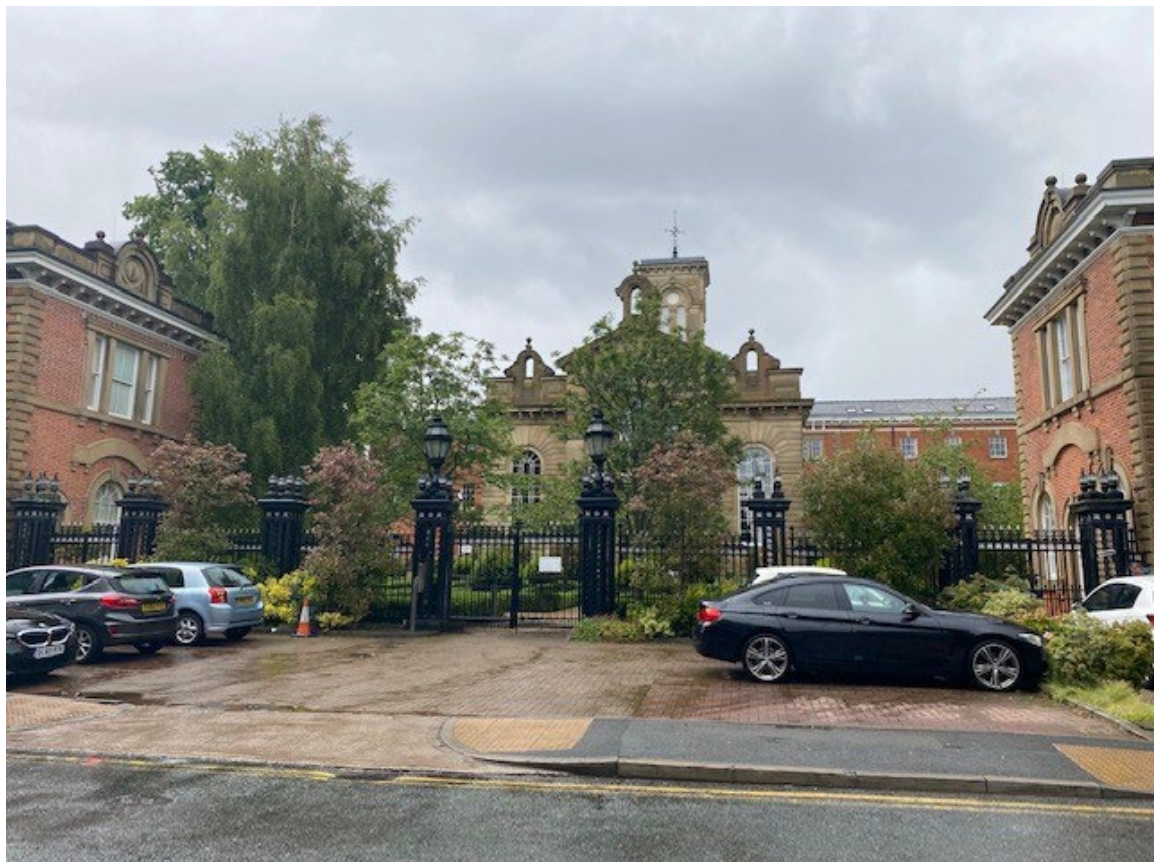
Figure 4.8 - Withington Hospital (Principal Administrative Block), view looking north. (Source: Author, 2022)
