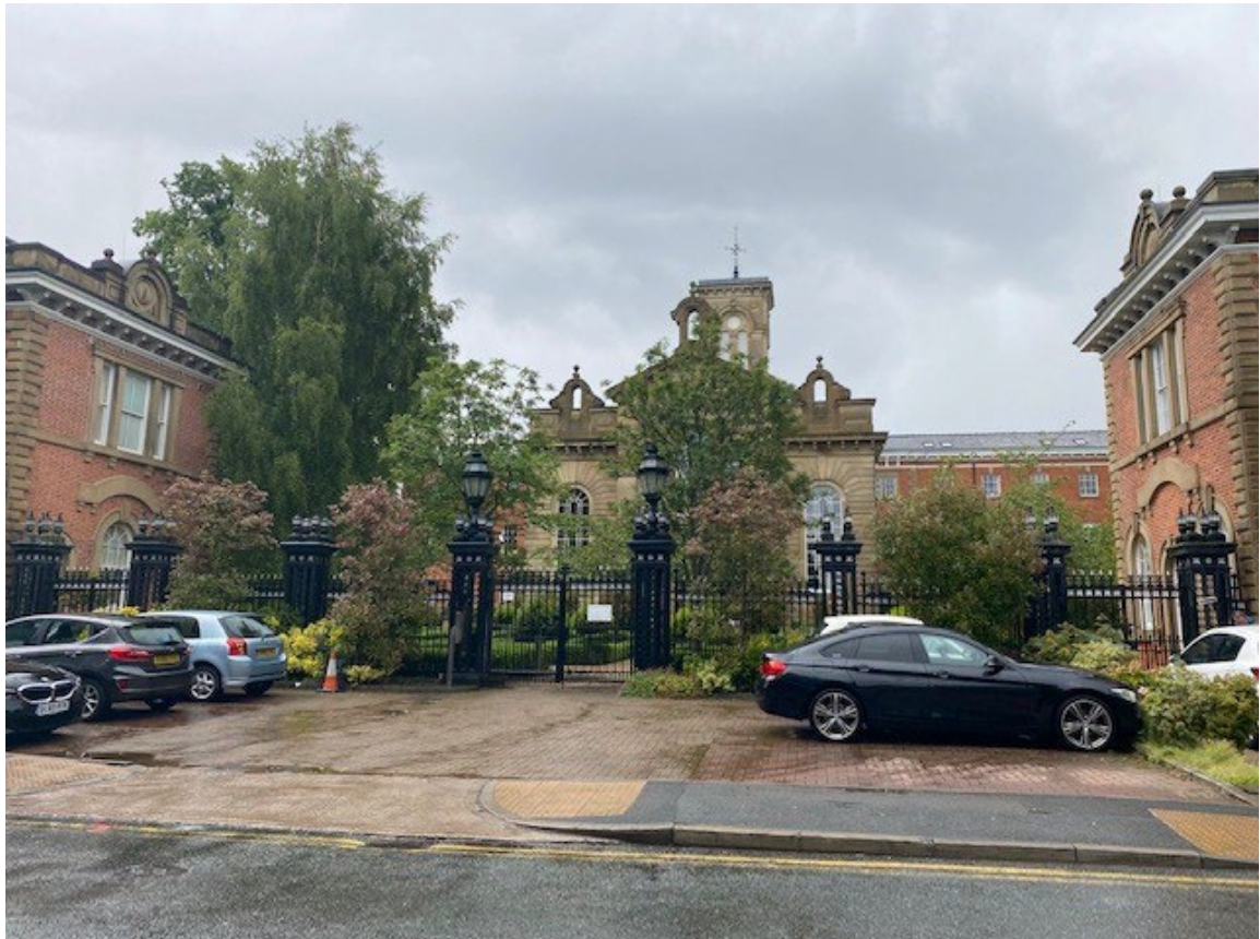
Figure 6.7 - Withington Hospital (Principal Administrative Block), view looking north. (Source: Author, 2022)
