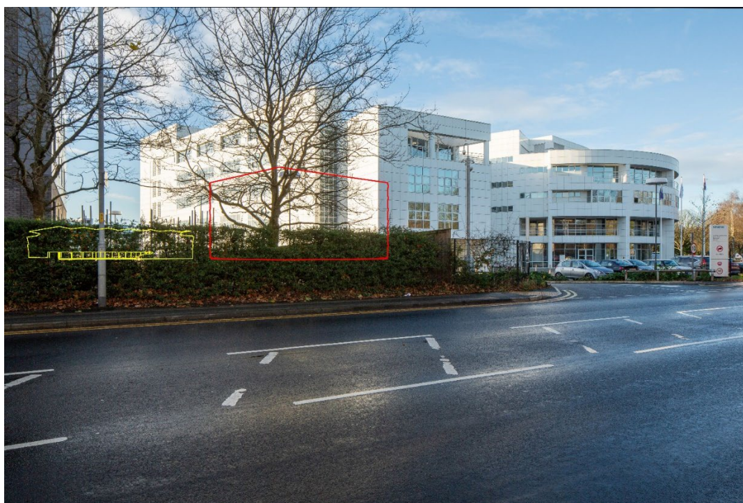
Figure 6.8 - Withington Hospital (Principal Administrative Block), view looking north. (Source: Our Studio, 2022, marked up by Deloitte)
