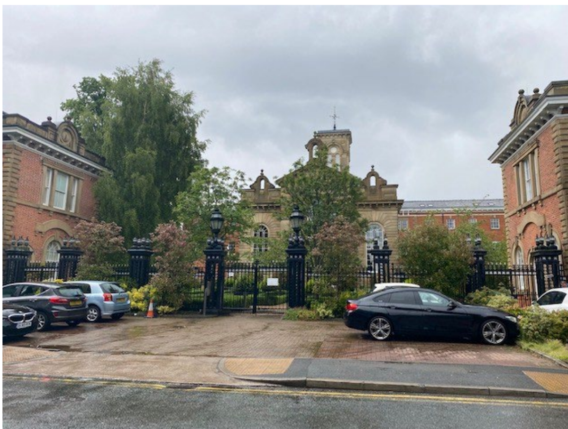
Figure 5.13 - Withington Hospital (Principal Administrative Block), view looking north. (Source: Author, 2022)
