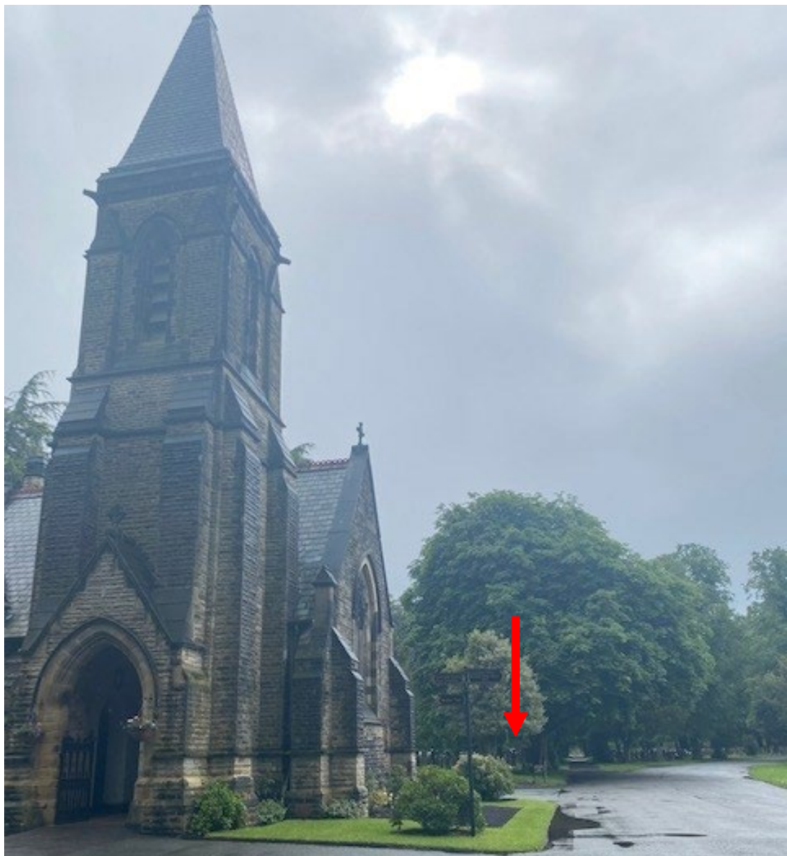
Figure 4.5 – Photo of Church of England Chapel , view looking east. Approximate Site location indicated by red arrow. (Source: Author, 2022)
