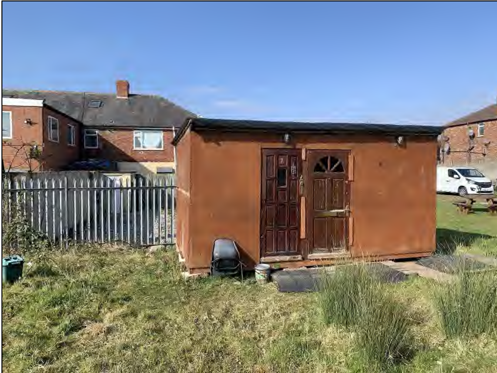
Plate 9 – The single building present on site, anecdotally understood to be used as a toilet block
