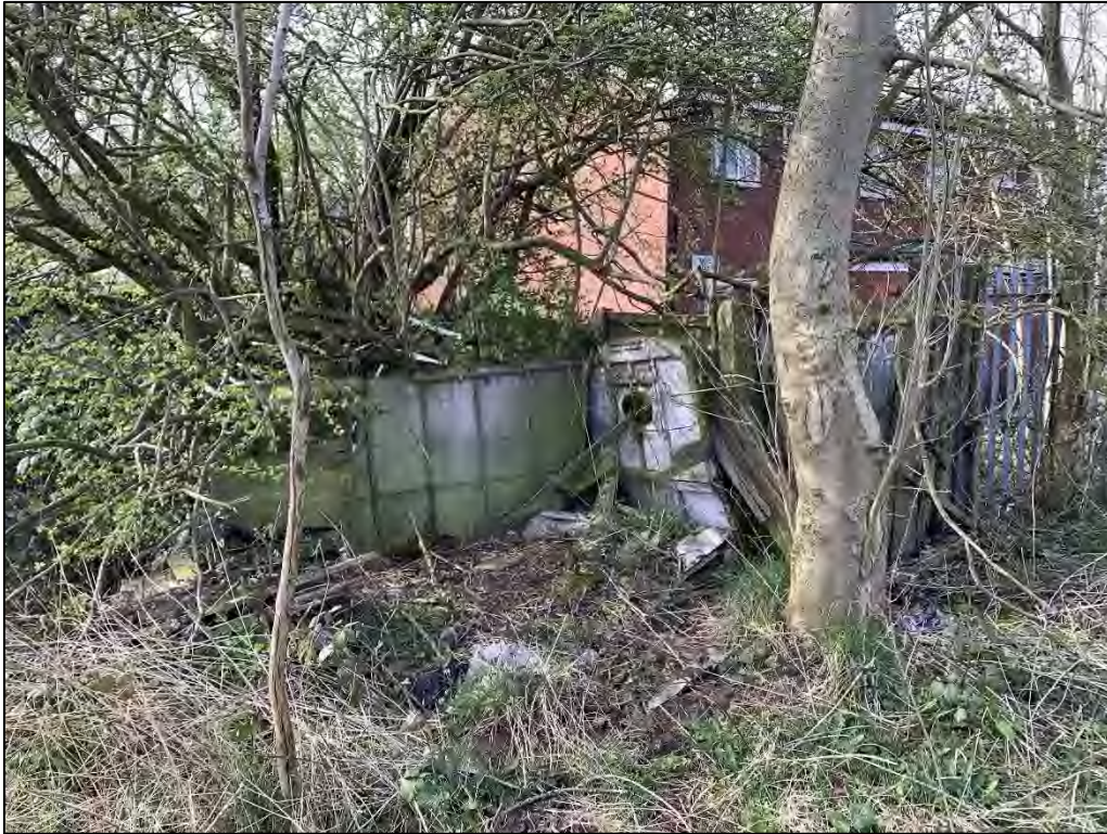
Plate 15 – Further angle of the southern boundary, showing the dilapidated nature of the fence
