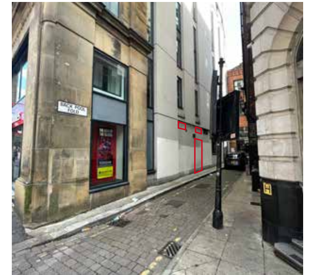
VIEW OF DOOR & GRILLE LOCATION FROM CROSS ST.
