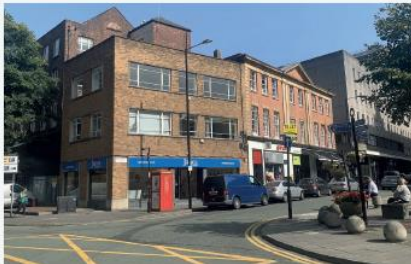
Existing buildings at 27-29 King Street West (left) and Reedham House (right).
