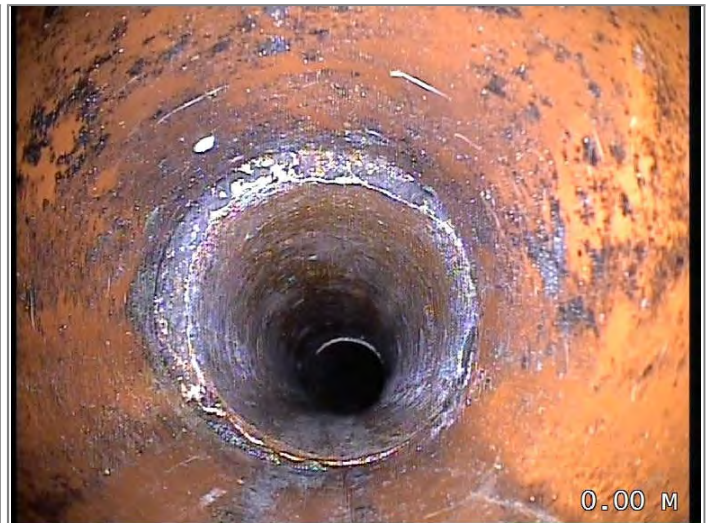
Water level 5% height/diameter
