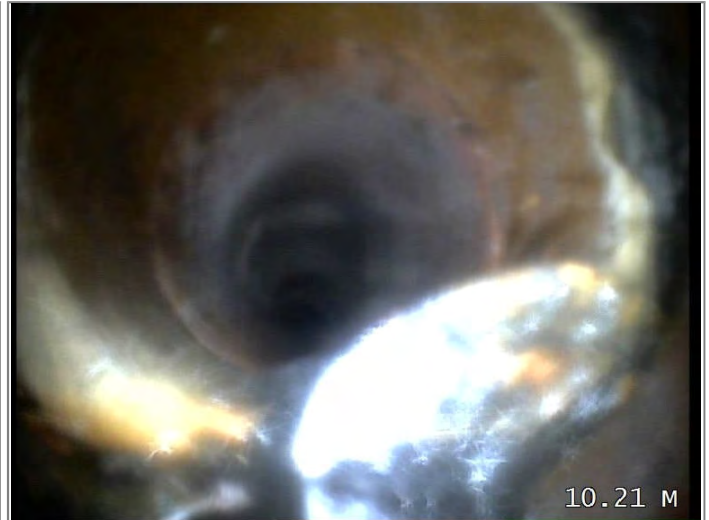
Survey abandoned - Remark: UNABLE TO PASS DUE TO DISPLACED JOINT - ENCRUSTATION - REPAIR NEEDED
