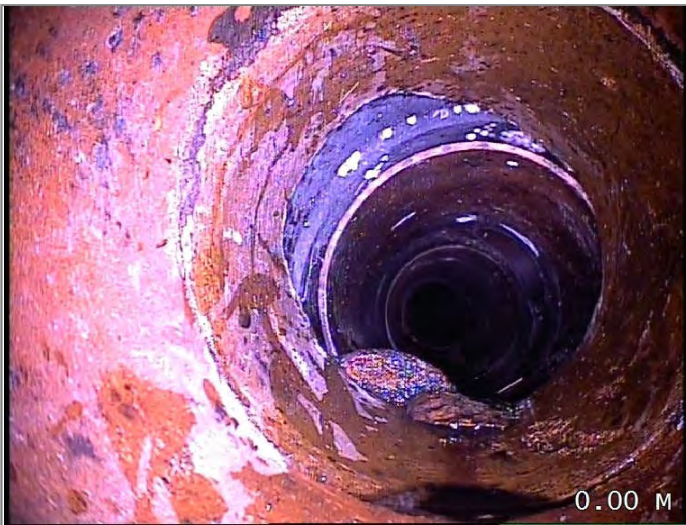
Start node type, manhole, reference MH 02
