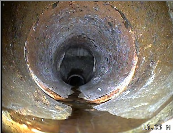
Material of drain/sewer changes to vitrified clay at this point
