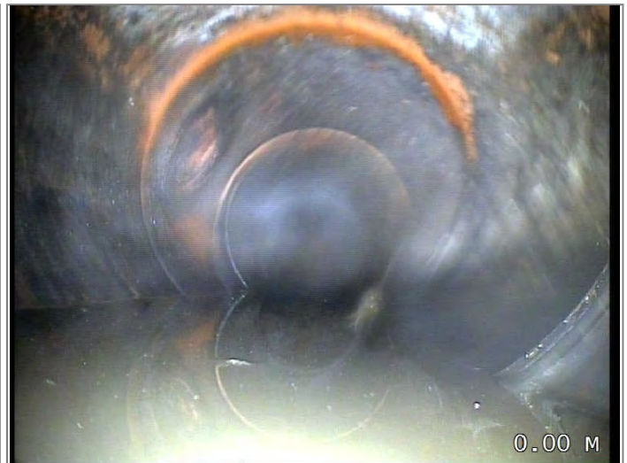
Water level 10% height/diameter
