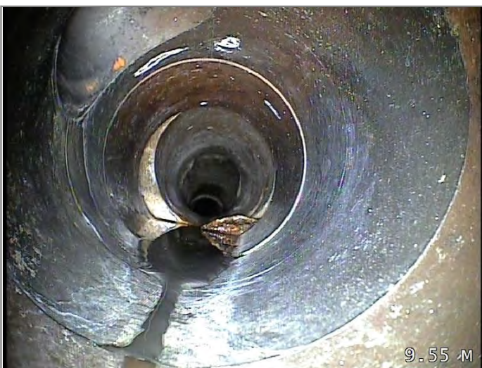
Junction at 10 o'clock, diameter 100mm
