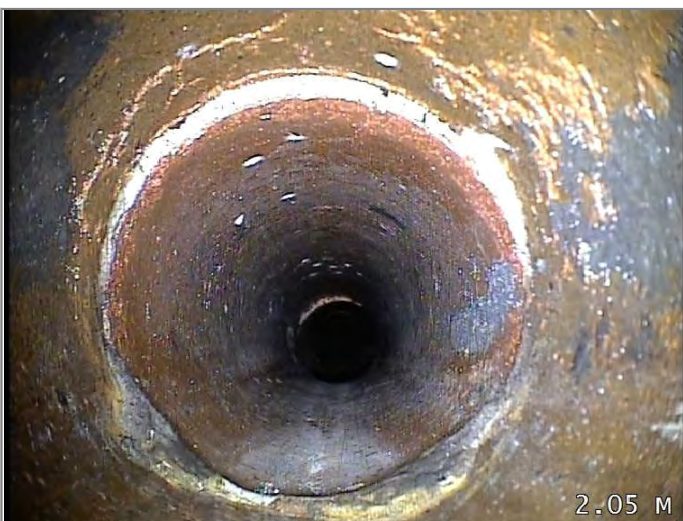
Attached deposits, encrustation from 4 to 8 o'clock 5% cross-sectional area loss
