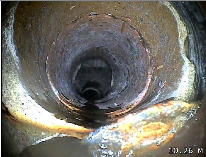
Attached deposits, encrustation at 5 o'clock 5% cross-sectional area loss
