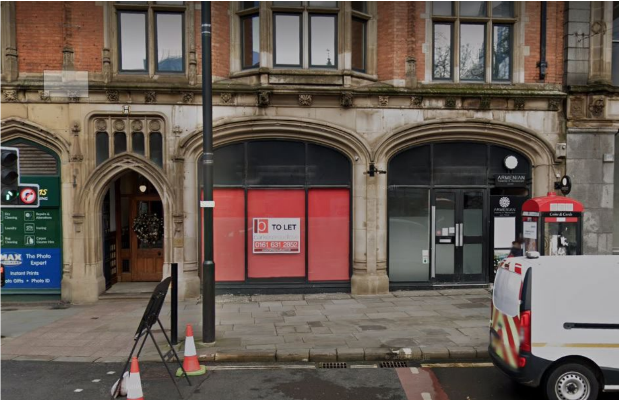
Existing shop front within the two arches
