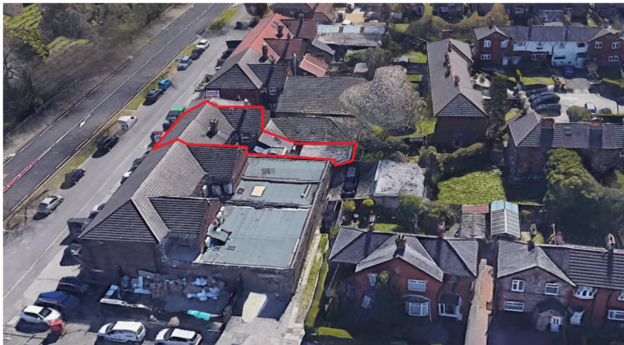
View eastwards with application site edged red and residential properties to the right
