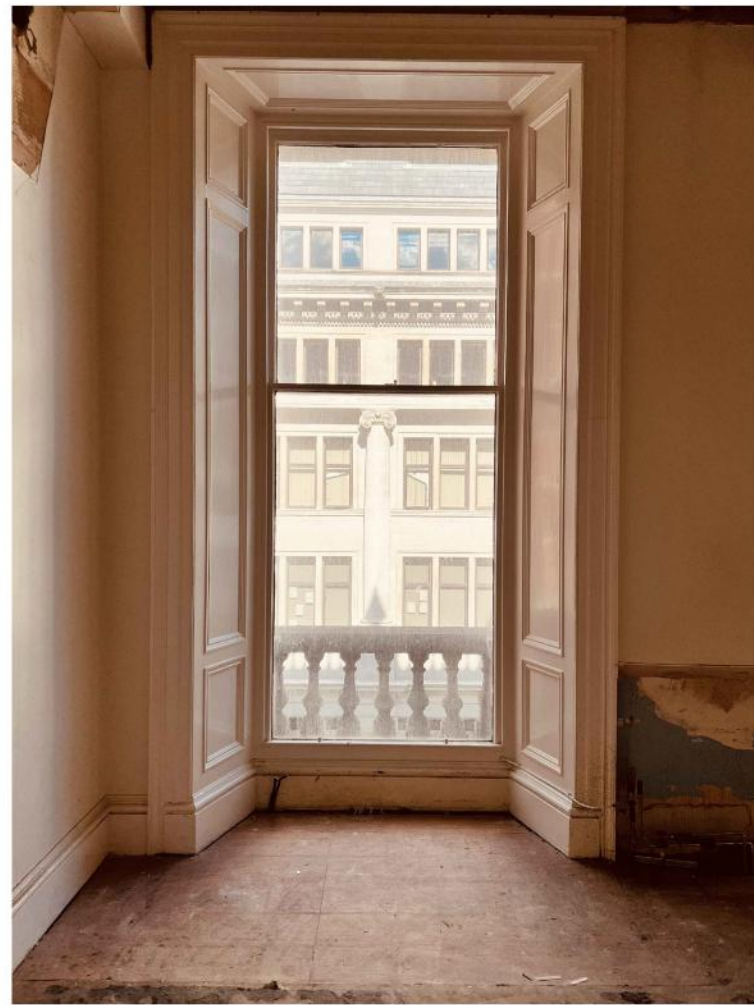
03 SECOND FLOOR EXISTING WINDOW PHOTO 576 SCALE - N/A PHOTOGRAPH
