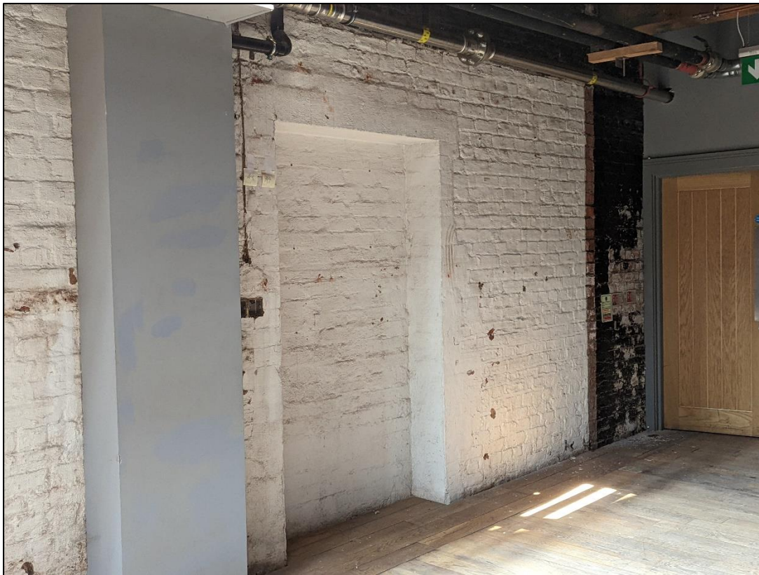
Plate 39: Blocked doorway in east wall
