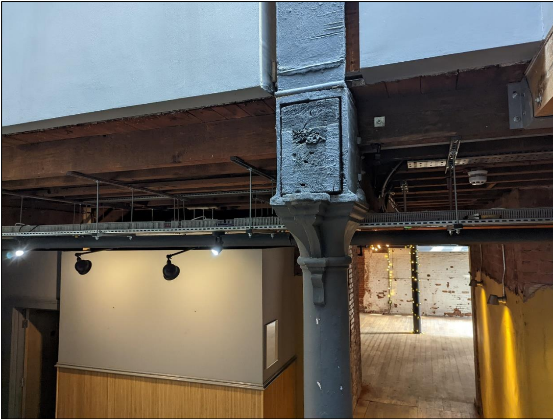
Plate 29: Detail of cut off beam for staircase insertion
