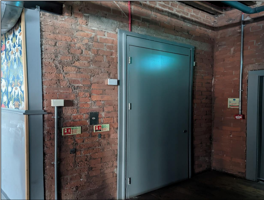
Plate 27: Original hoist shaft
