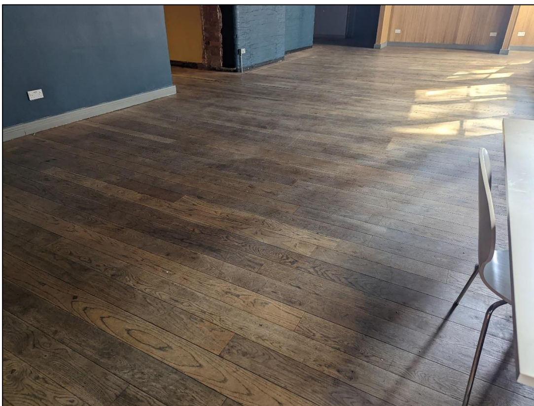
Plate 14: Detail of original boards
