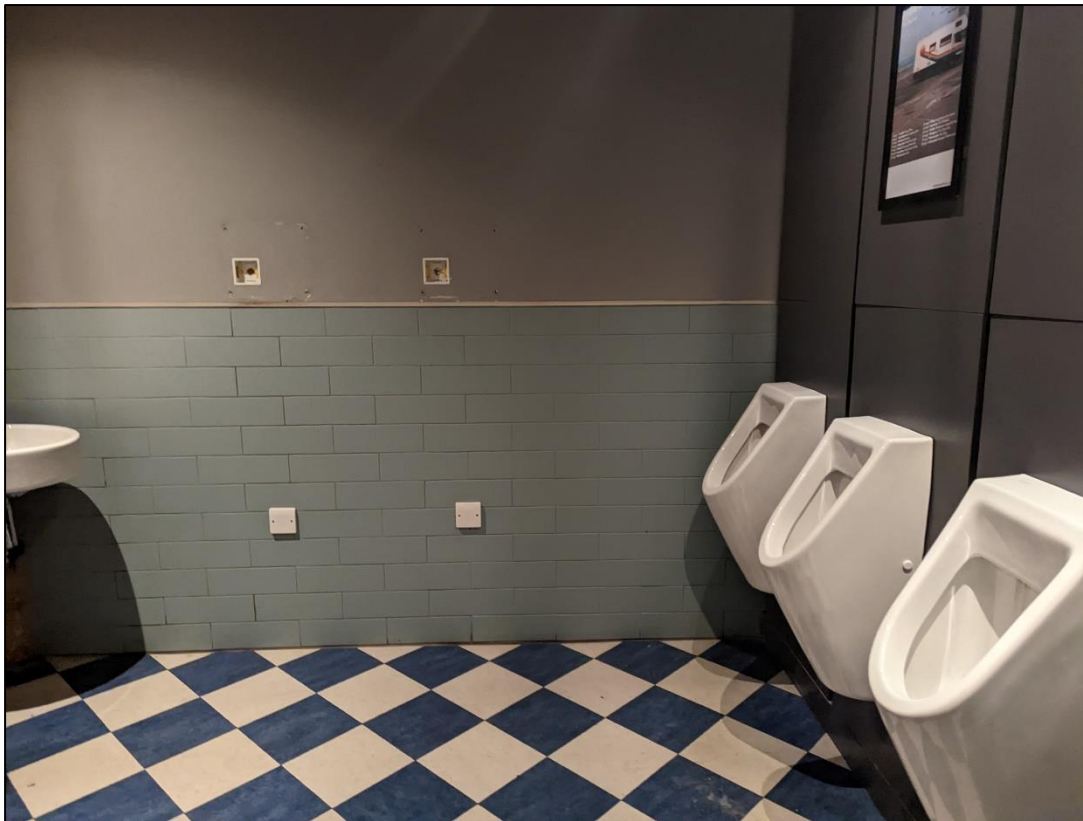
Plate 31: Inserted toilets to basement
