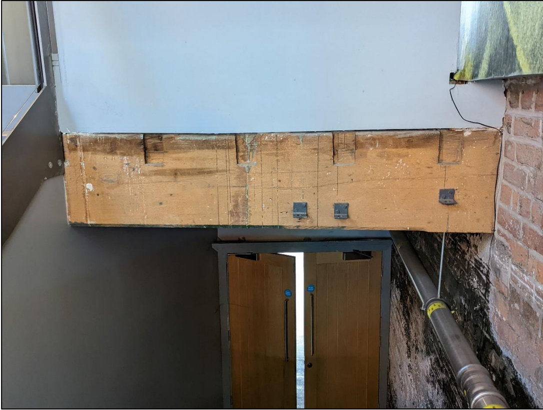
Plate 41: Removed joists for staircase insertion
