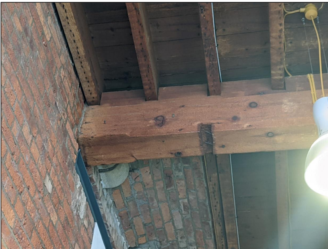
Plate 12: Ceiling detail showing timber joists and chamfered and stopped timber beams
