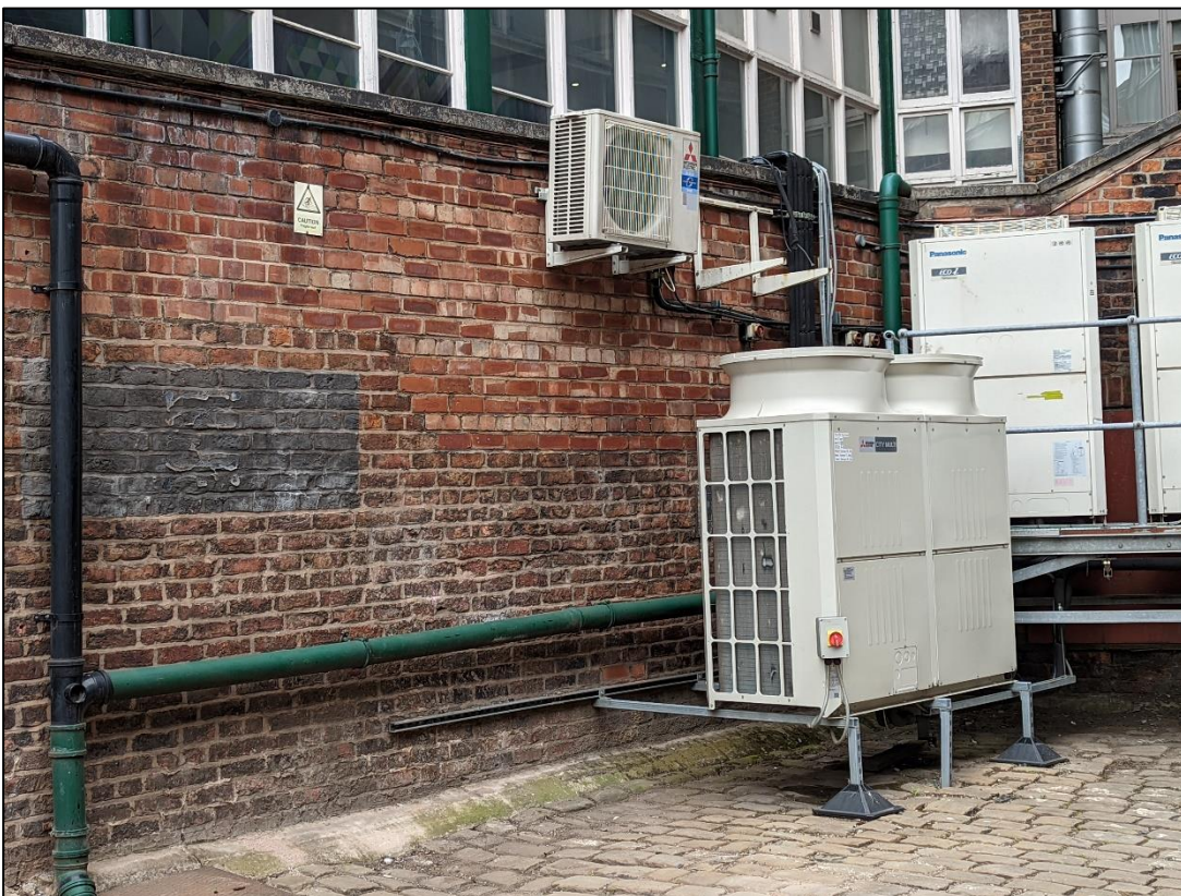
Plate 8: Boundary wall showing rebuild
