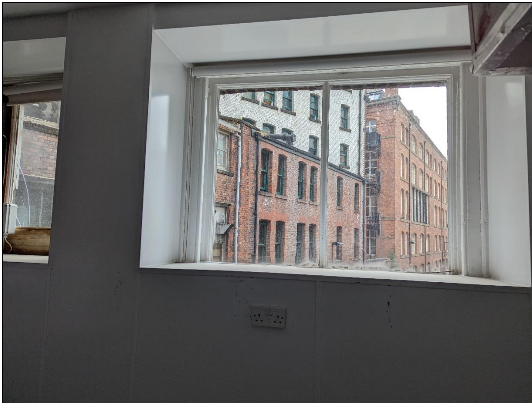
Plate 25: Windows in kitchen with original glazing
