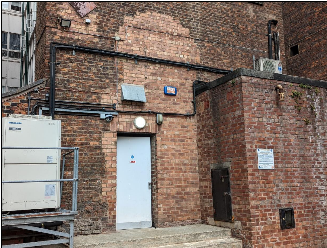
Plate 5: South elevation showing inserted doorway within blocked loading doorway
