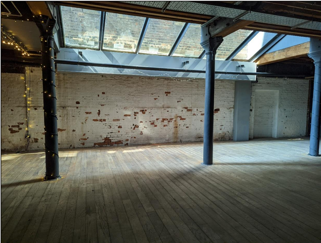
Plate 34: Western end of basement showing lightwell
