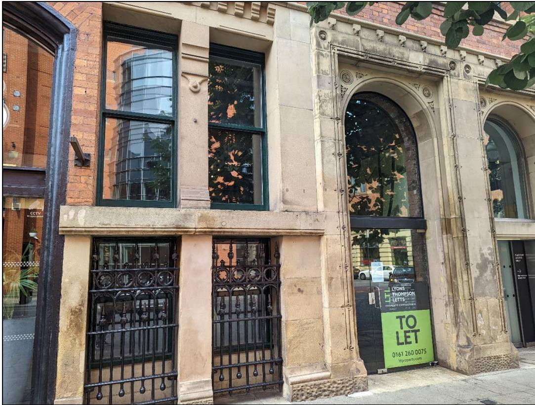
Plate 3: Ground floor of north elevation, bays 5 & 6
