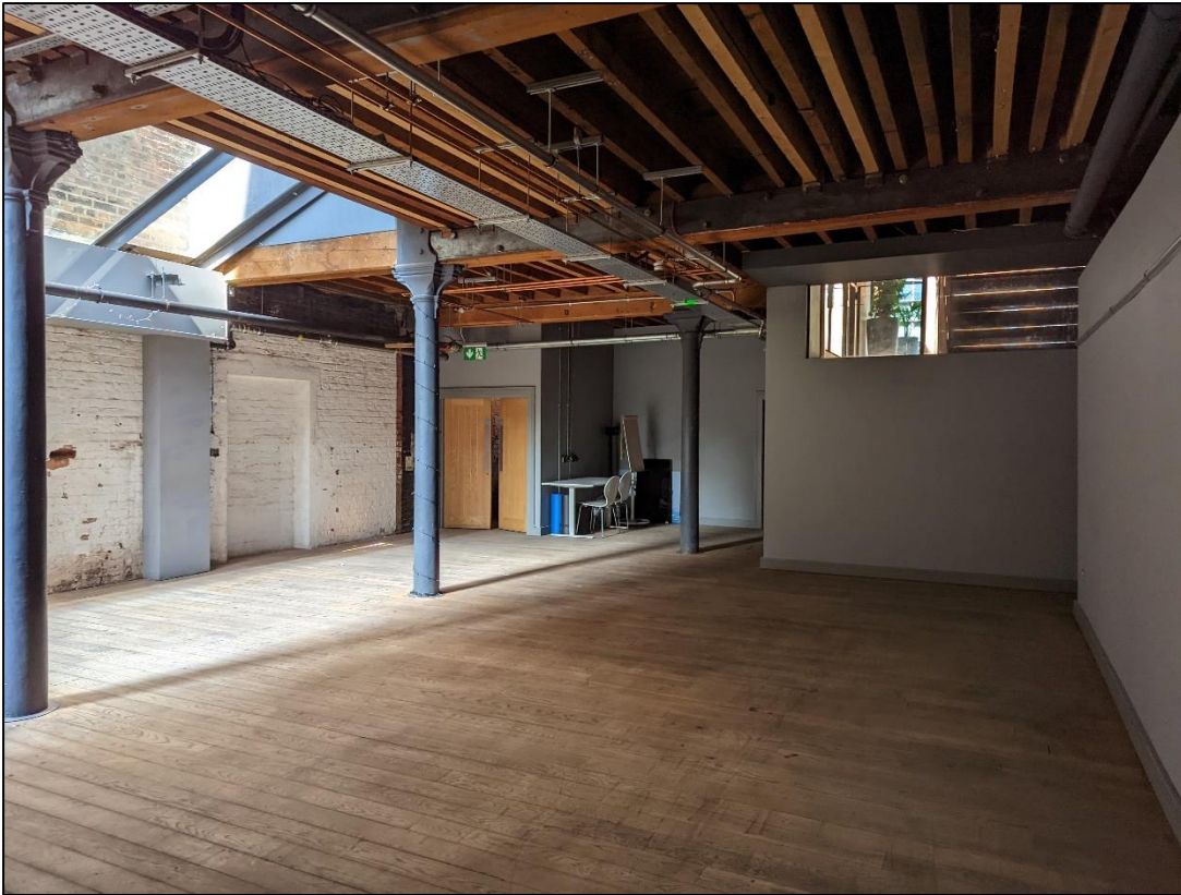
Plate 37: Area of inserted timber supporting joists
