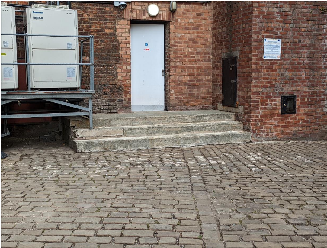
Plate 7: Inserted doorway with concrete steps up
