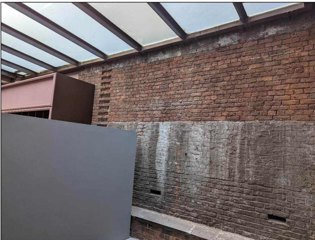
Plate 20: Bare brick eastern wall showing scar
