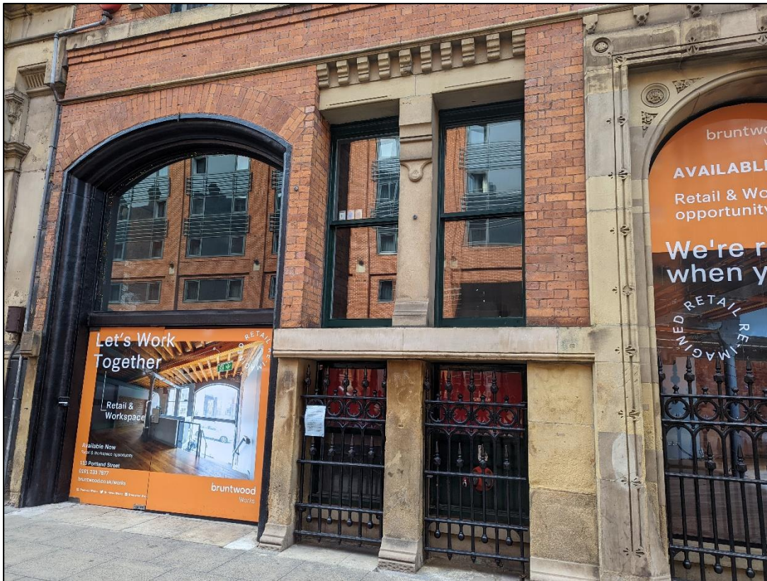
Plate 1: Ground floor of north elevation, bays 1 – 3
