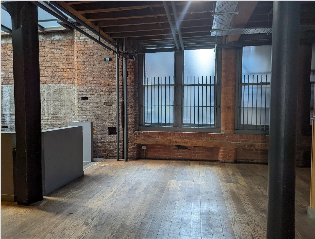
Plate 19: Windows in south end of east wall
