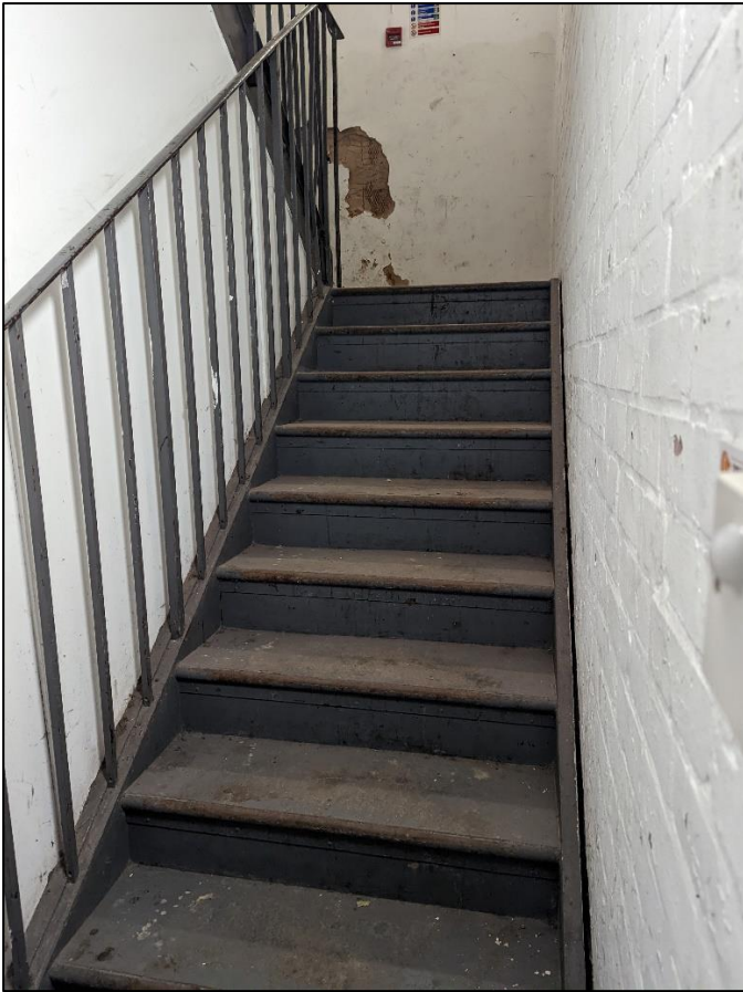
Plate 33: Rear fire escape staircase
