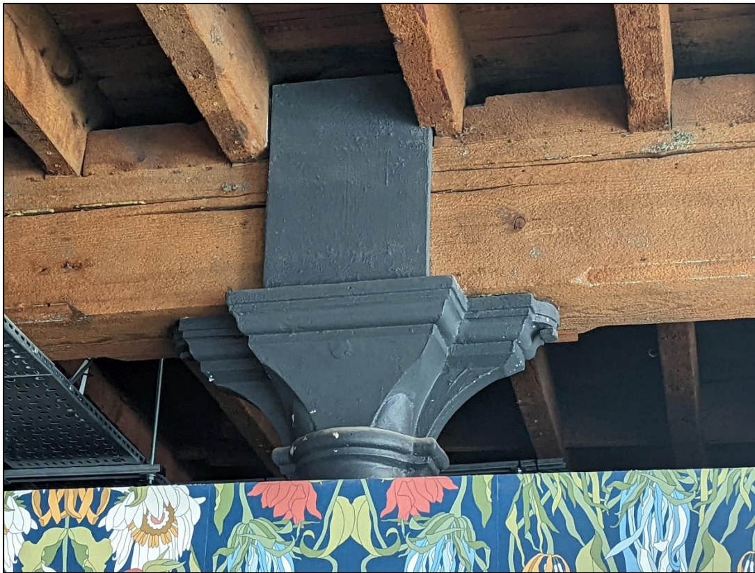
Plate 17: Detail of stanchion capital
