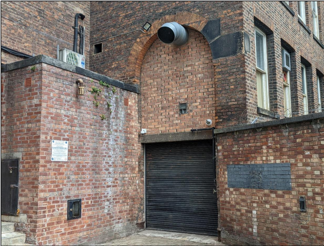
Plate 9: Loading Bay entrance in west elevation to rear yard
