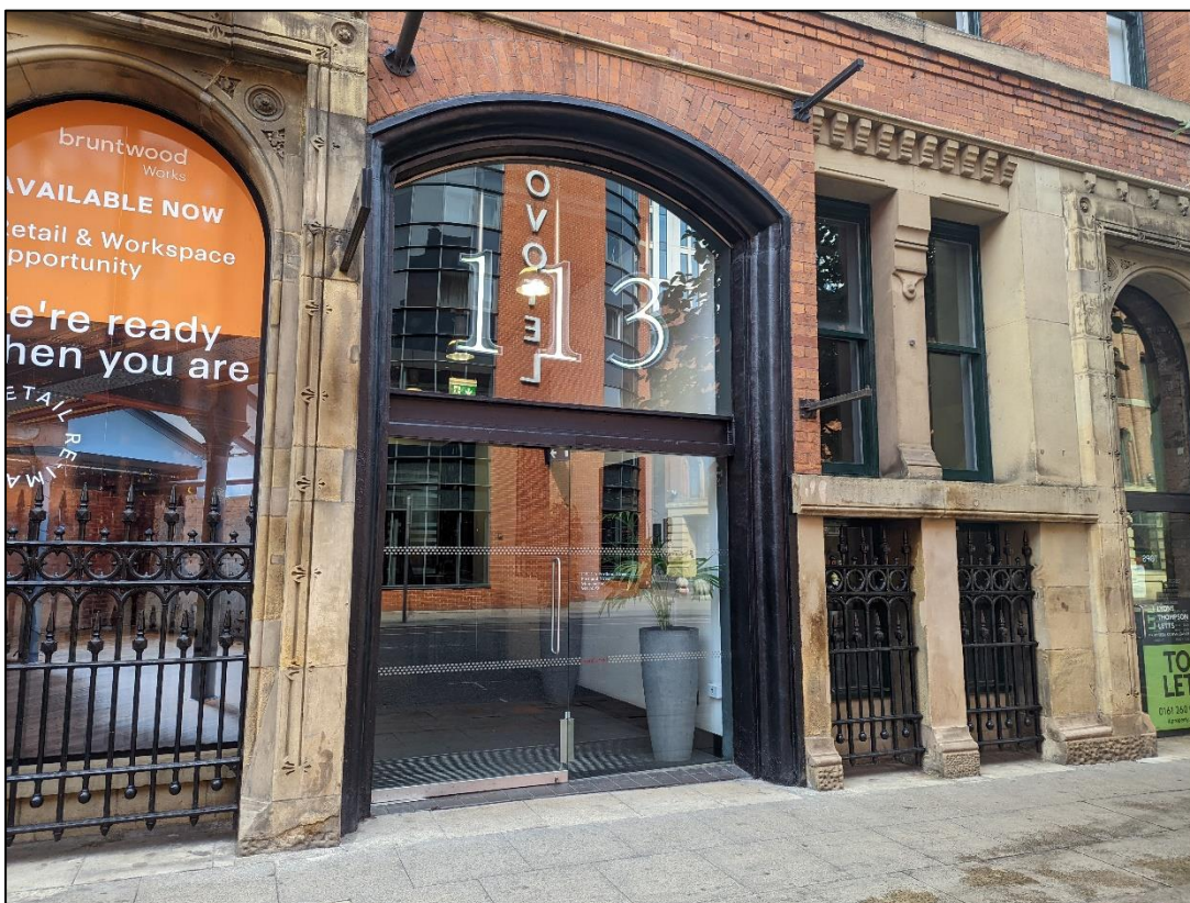
Plate 2: Ground floor of north elevation, bays 3 - 6
