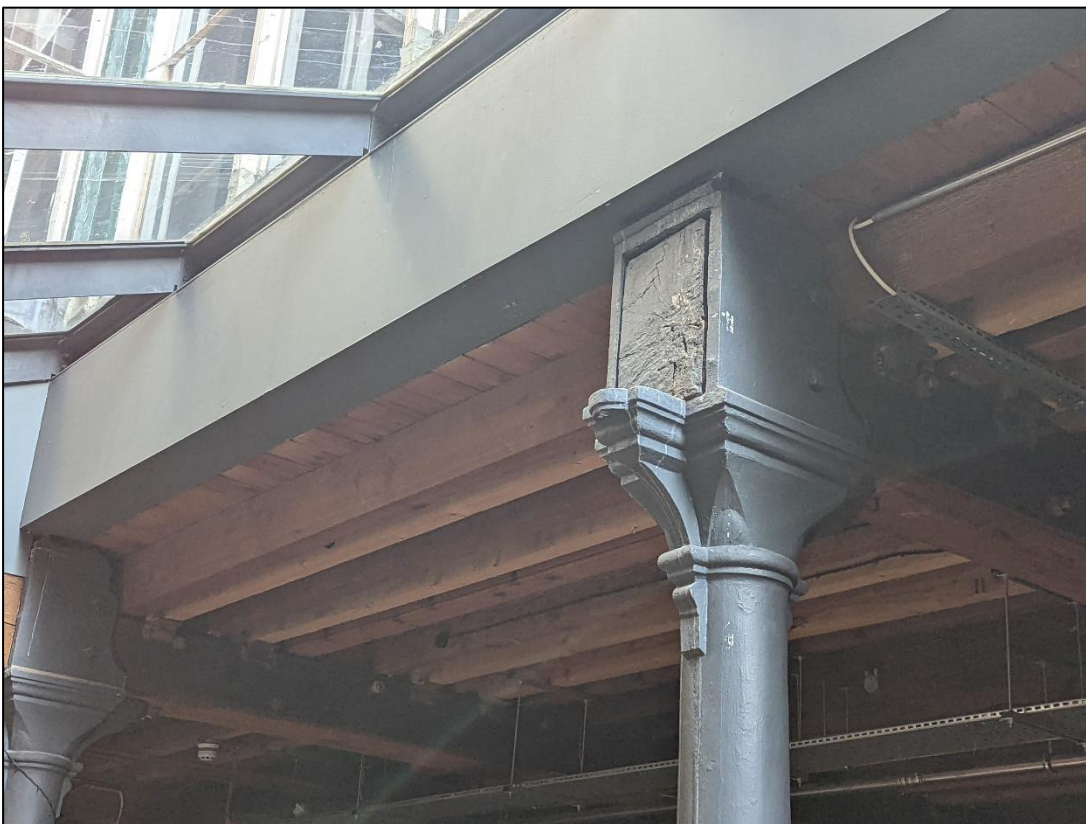
Plate 36: Cut off beam across light well
