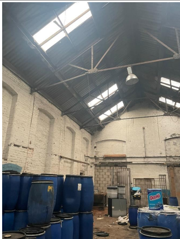
Figures 55 and 56: early 20 th century extension to casting & pattern store. Looking east into later extension to workshop. The interior has been compromised by modern interventions and loss of historic features; metal trusses remain
