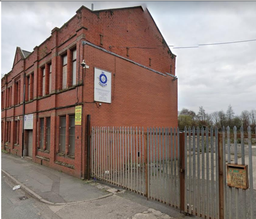
Figure 32: early 20 th century extension to office range (north elevation): Principally blank gable with pitched roof detail evident. Protective gate and signage all of a later date.
