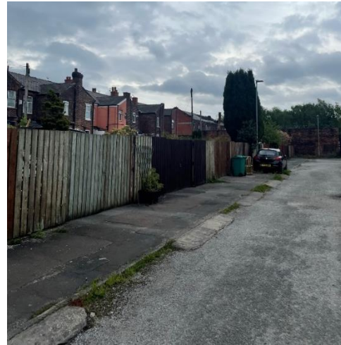
Figure 60: Rear side to housing, Ferris St. Some of the dwellings to this street have been lost.
