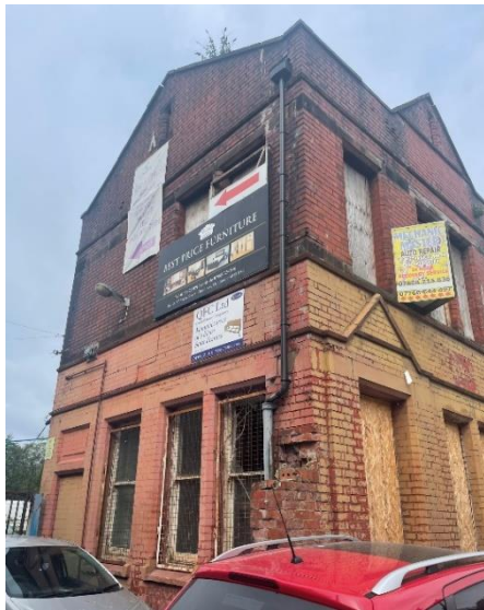
Figure 29 (left): Original office range (south elevation), designed c.1892. Two-storeys in red brick, flemish bond. Original window frames survive to ground floor (overcovered with protective metal barrier). Rainwater goods and signage are all later additions. Figure 30 (right): Rear elevation to original office range (east elevation). four bay section – more domestic in character; bays 11 & 10 with single windows / door – bay 9 with paired windows – bay 8 blank – bay 7 terminates in gablet over (badly damaged), above loading door and remnant of hoist beam – brick with brick-arched window heads, red-sandstone cills; projecting party wall between seven- and four-bay sections; windows and doors replaced. Original chimney survives, other has been lost.
