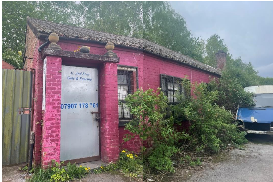
Figure 46: Small Workshop - North / Front elevation: Single-storey in height with a pitched corrugated (possible asbestos) roof; original window openings; porch later incongruous addition; chimney to west end; red brick with red sandstone heads and cills; windows and doors replaced; façade painted
