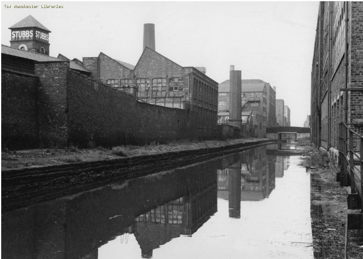
Figure 12: Ashton Line Canal view with Joseph Stubbs Mill Works in Ancoats visible to the left. Note the distinctive saw tooth roof and 'STUBBS' branding to all faces of the stair tower. Source: Manchester Image Archive, ref: m53855
