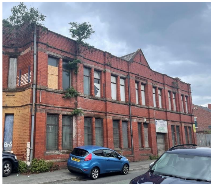
Figure 31: early 20 th century extension to office range: Two-storeys in height with a pitched roof set behind a parapet; composed in two sections of seven bays respectively; seven bay section advanced to back of
