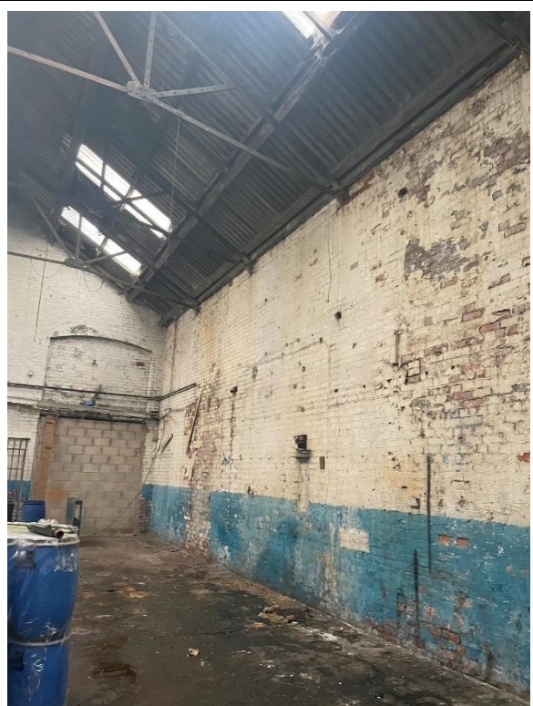
Figures 55 and 56: early 20 th century extension to casting & pattern store. Looking east into later extension to workshop. The interior has been compromised by modern interventions and loss of historic features; metal trusses remain
