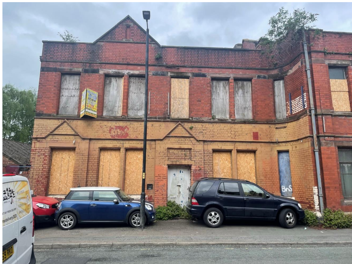
Figure 28: Original office range – Principal (east) elevation, designed c.1892. Two-storeys in red brick, flemish bond. Simple stone banding above ground floor and first floor windows. Simple parapet detail. One chimney survives. Windows overcovered with boarding. REEFER TO FIGURE 18 ABOVE FOR DETAIL OF ORIGINAL OFFICE RANGE AS DESIGNED IN 1892.
