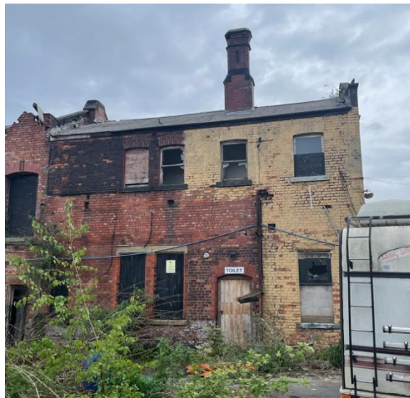
Figure 29 (left): Original office range (south elevation), designed c.1892. Two-storeys in red brick, flemish bond. Original window frames survive to ground floor (overcovered with protective metal barrier). Rainwater goods and signage are all later additions. Figure 30 (right): Rear elevation to original office range (east elevation). four bay section – more domestic in character; bays 11 & 10 with single windows / door – bay 9 with paired windows – bay 8 blank – bay 7 terminates in gablet over (badly damaged), above loading door and remnant of hoist beam – brick with brick-arched window heads, red-sandstone cills; projecting party wall between seven- and four-bay sections; windows and doors replaced. Original chimney survives, other has been lost.
