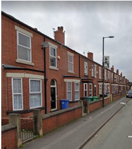
Figure 59: Purpose built workers housing (designed c.1899 by J. Nodal for Joseph Stubbs).
