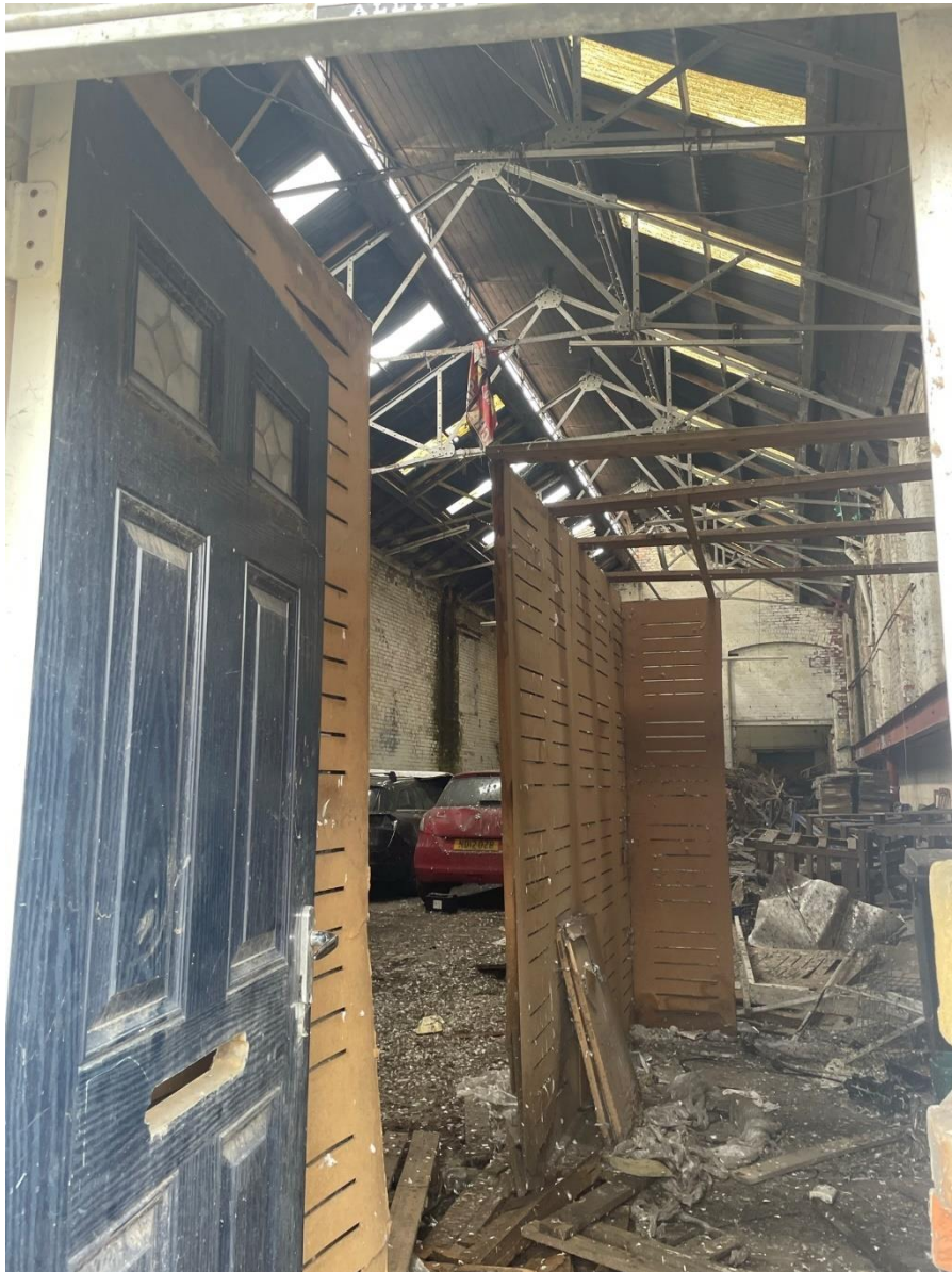
Figure 54: View into original late 19 th century workshop space from alleyway. Some discernable features such as the lantern roof and trusses survive. There is little tangible evidence (fixed machinery etc.) which indicates the workshop was a purpose built casting store.
