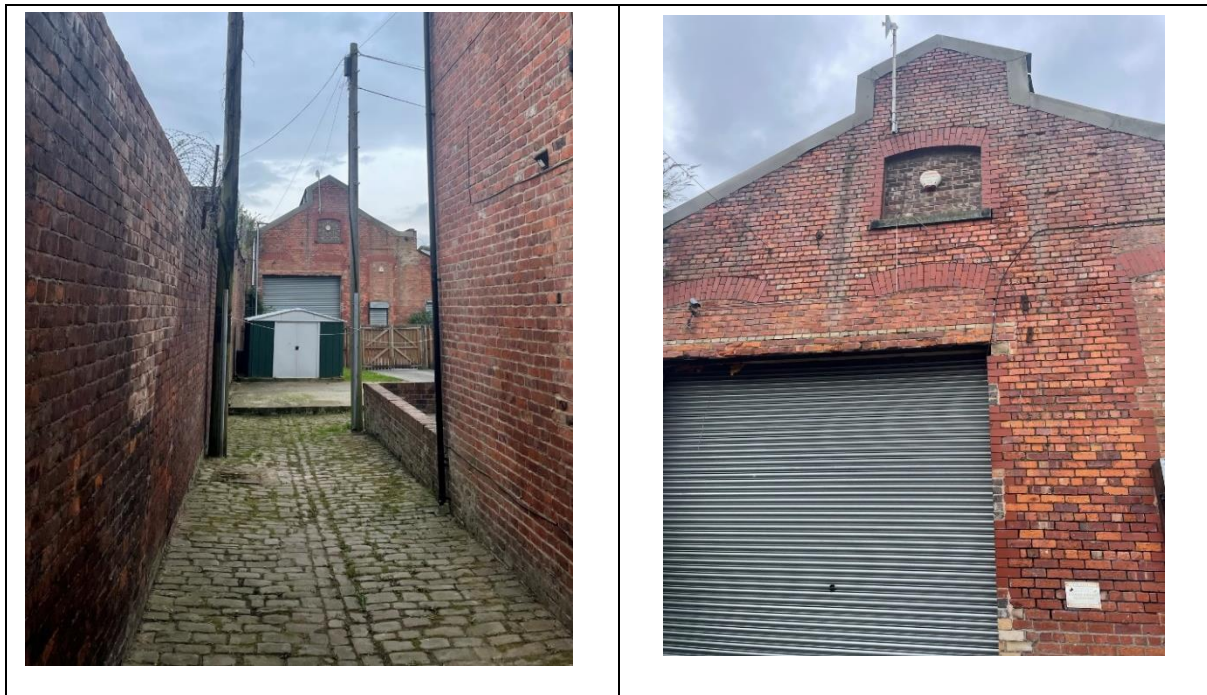
Figures 52 and 53: east elevation to original former casting and pattern workshop, as designed by J.Nodal.
