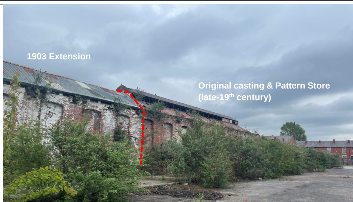
Building 4: Large workshop (former Casting & Pattern Store) - Exterior
