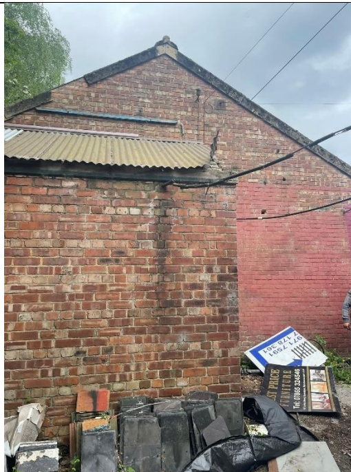
Figure 46: Small Workshop - North / Front elevation: Single-storey in height with a pitched corrugated (possible asbestos) roof; original window openings; porch later incongruous addition; chimney to west end; red brick with red sandstone heads and cills; windows and doors replaced; façade painted
