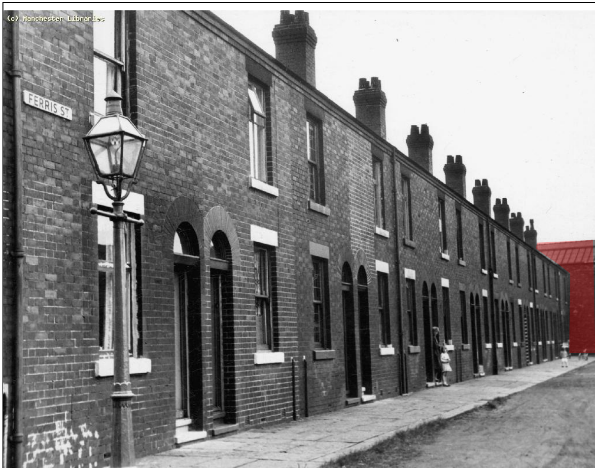
Figure 21 Openshaw, Ferris Street from Louisa Street, pictured c.1964. The mid-20 th century illustrates the late-19 th / early 20 th century terraced housing as built. Note the Iron Foundry is discernible to the far right of the image (shaded red). These have since been demolished. Source: Manchester Image Archive. Ref: m37227
