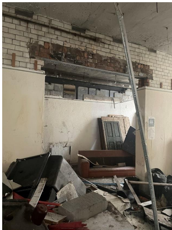
Figure 34: Ground floor to former office, looking north. Some evidence of early-20 th century brick wall in English bond. Modern plaster covering a number of features. Possible, original glazed screen to room beyond.
