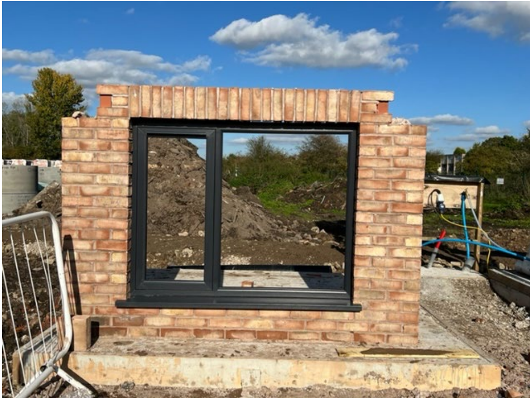
This is the new Flush fit casement window profile by linier which is slimmer to the one already specified
