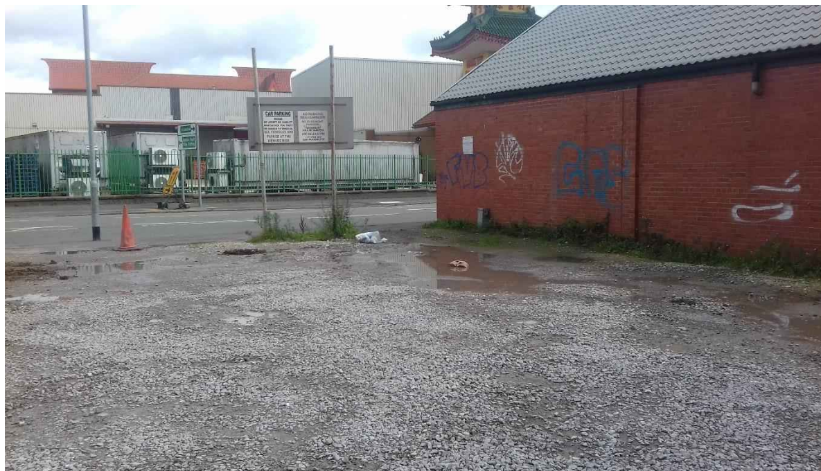
PLATE 2 VIEW OF EXISTING BUILDING
