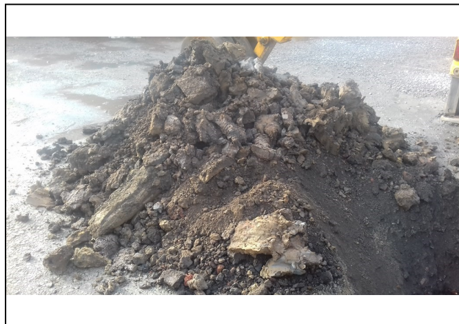
Trial Pit 101 Spoil
