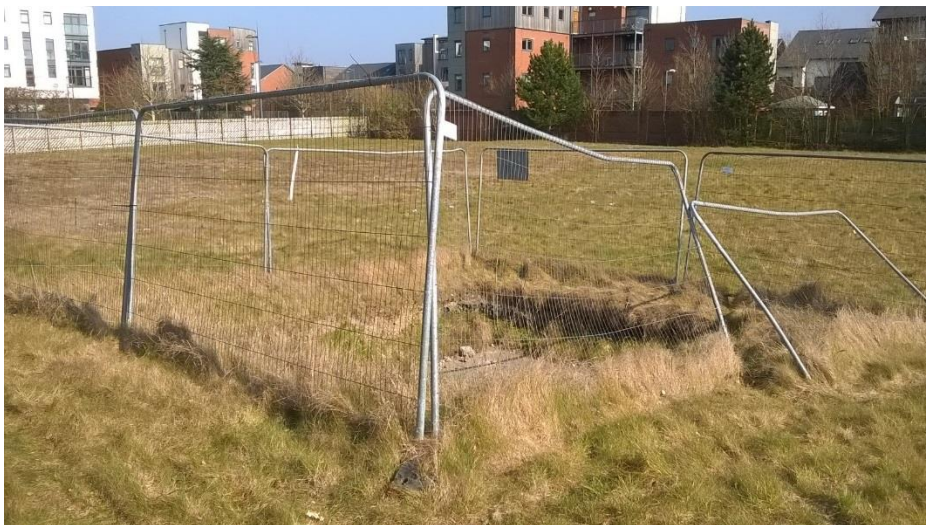
3) Buried slab, view looking north east
