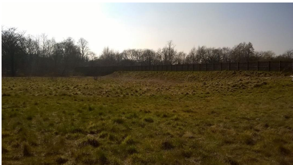
6) View looking south west showing elevated road.
