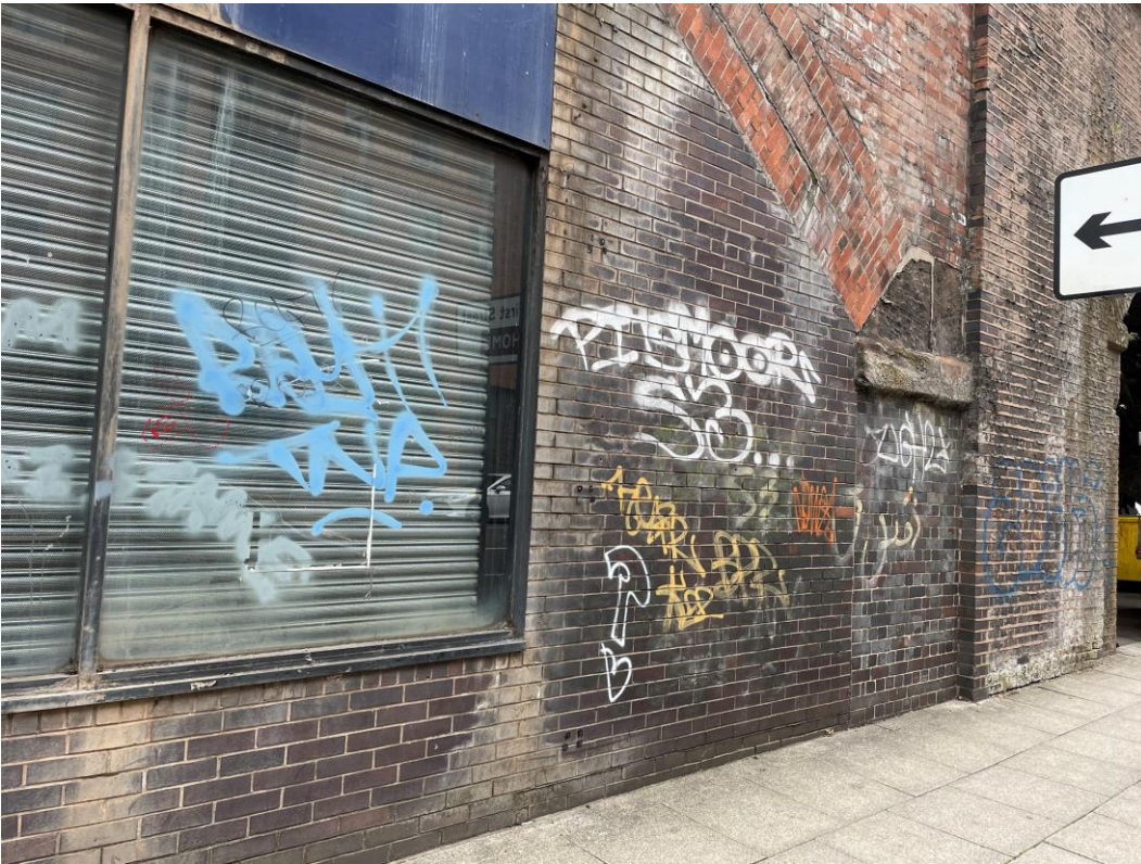
7) Right hand side of the brickwork infill where the proposed emergency exit would be situated.
