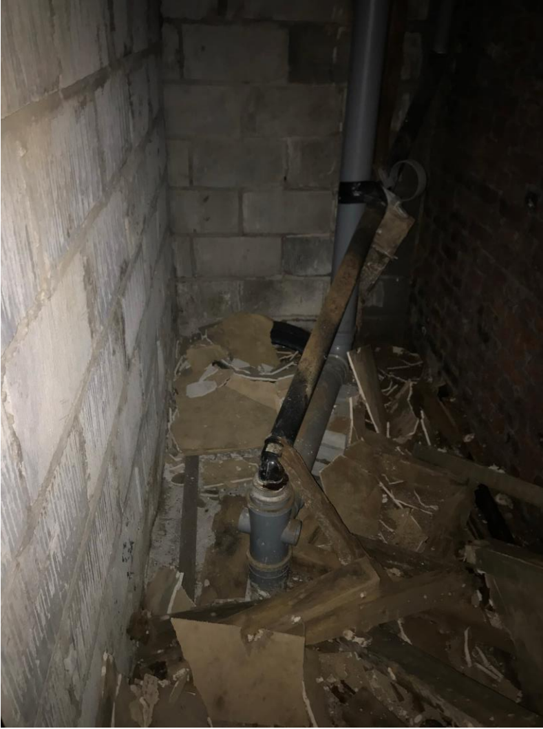
25) Debris to basement level. Location of existing foul waste which will be connected into as part of the WC construction works.
