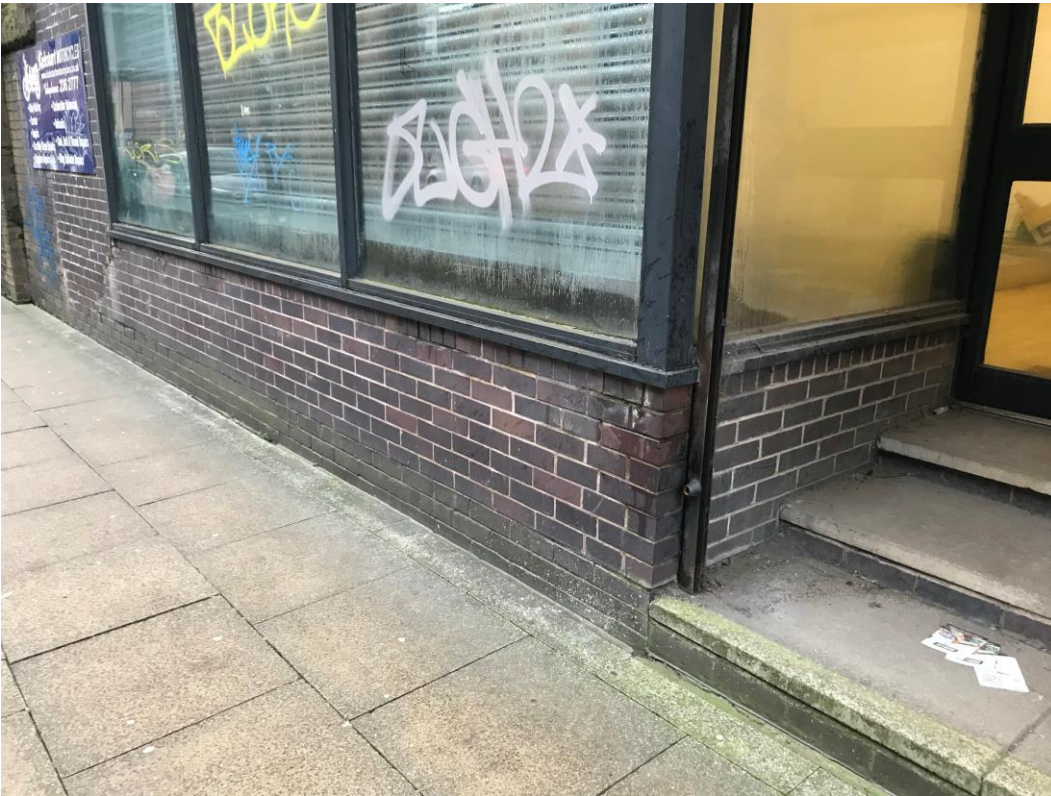
3) Left hand side soiled stall riser constructed using engineering brick.
