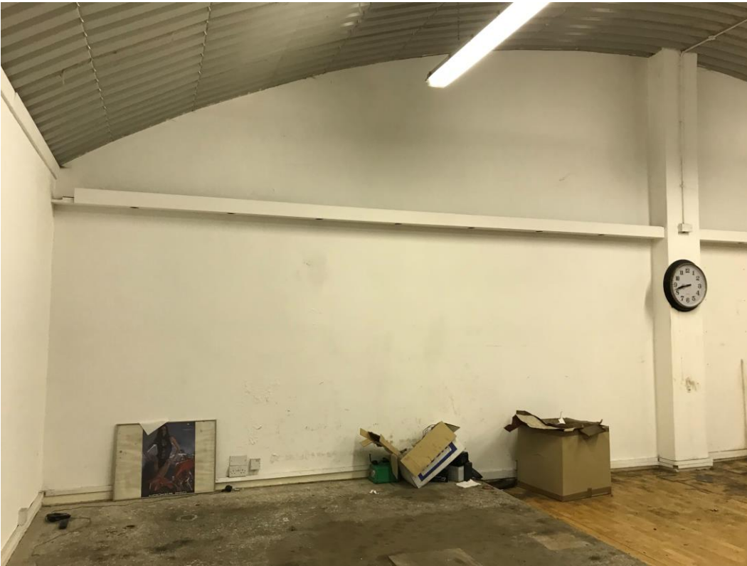
15) Overview of shop floor which has been formed from the existing mezzanine structure.
