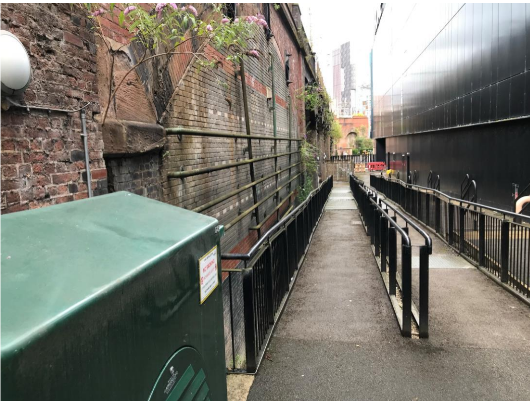
29) Overview of the rear infill with the neighbouring retaining structure in close proximity.
