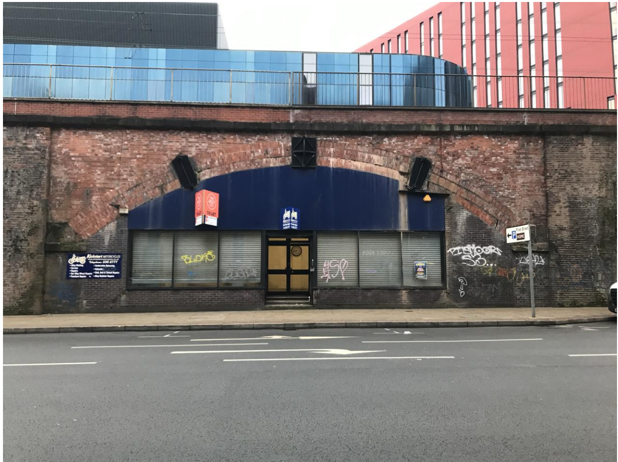
Figure 1 - Front elevation of the building
