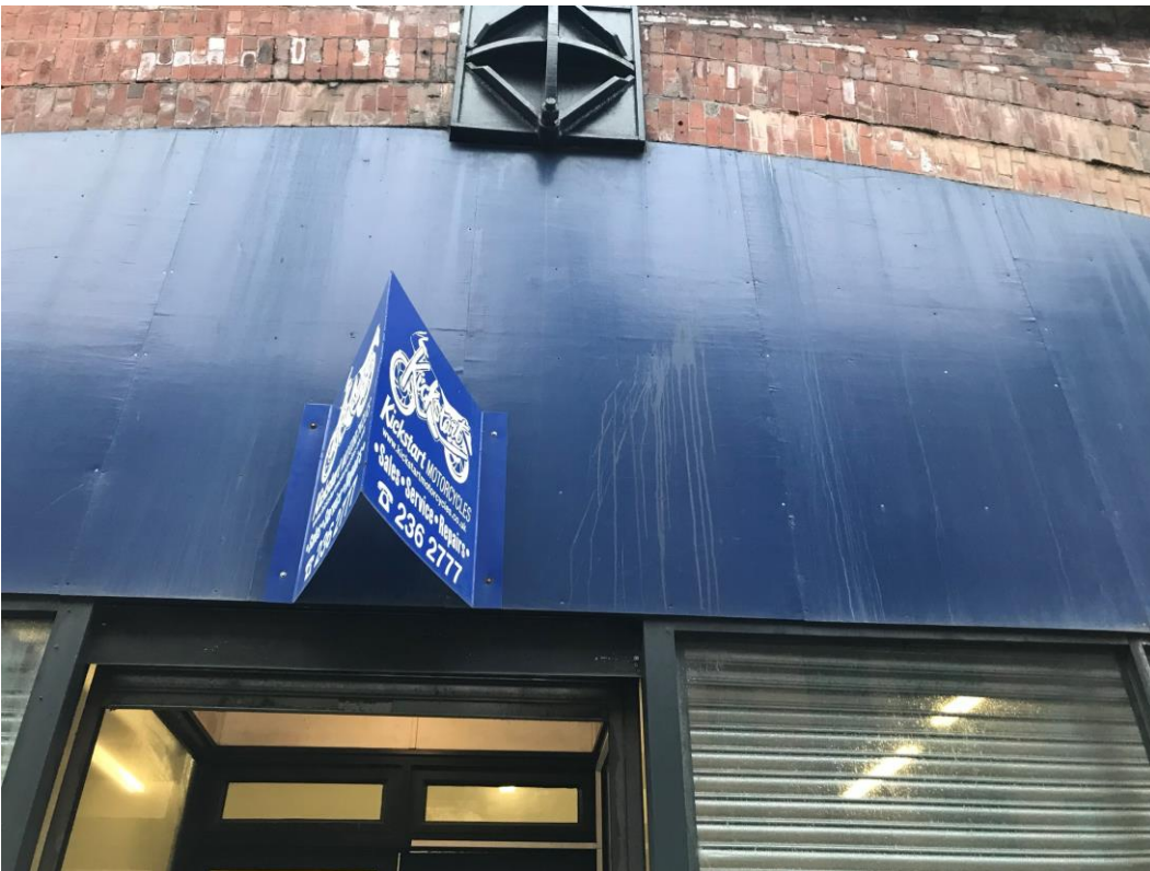
6) Painted signage fascia which would receive redecoration works as part of the project. The colour of paint would match the existing.
