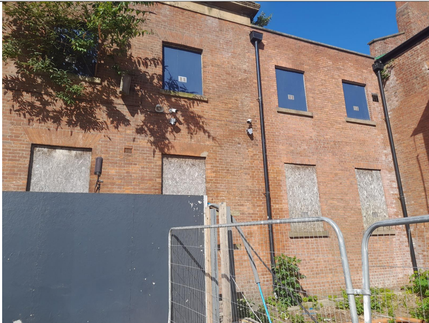
Existing buildings on site. Fenced off with Heras fencing to prevent access.
