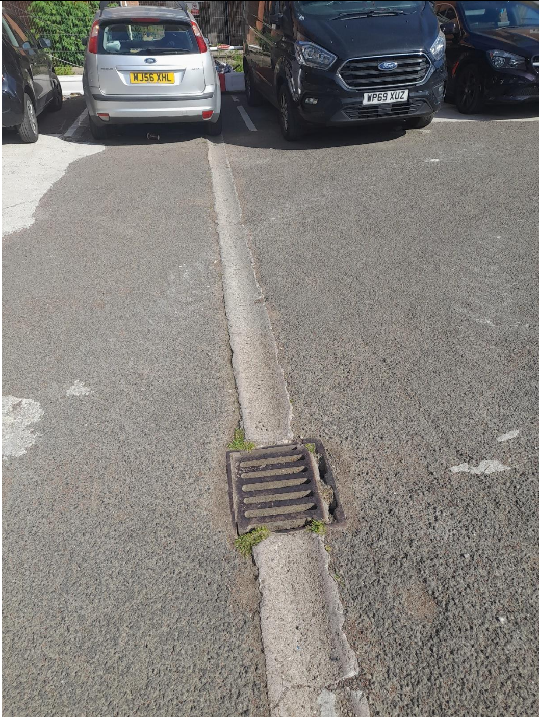
Surface drains noted on site.
