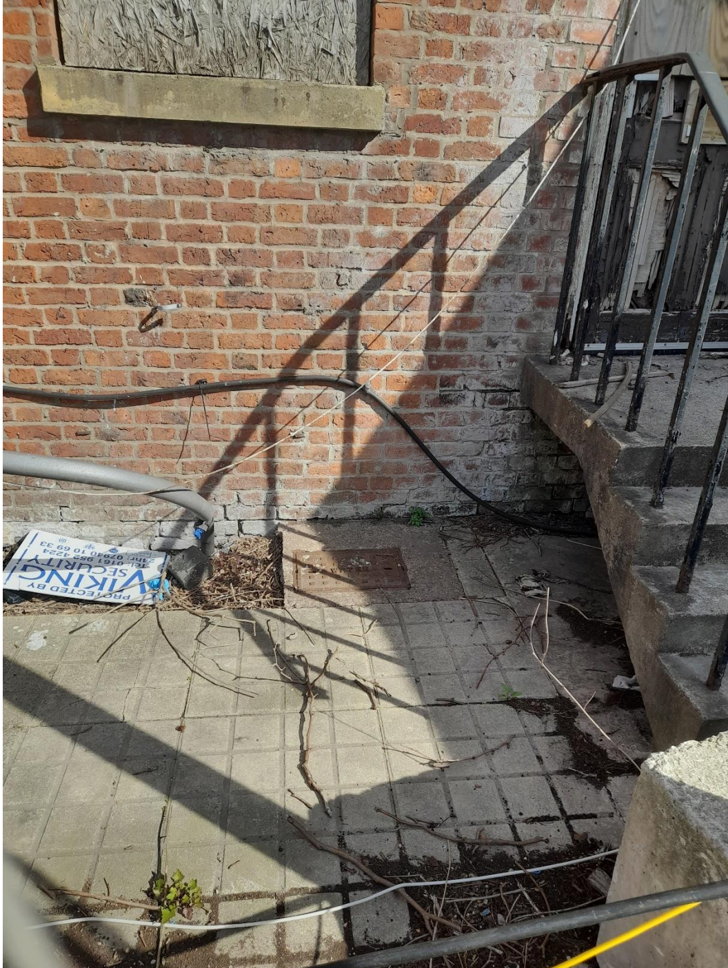
Services noted associated with existing building on site.
