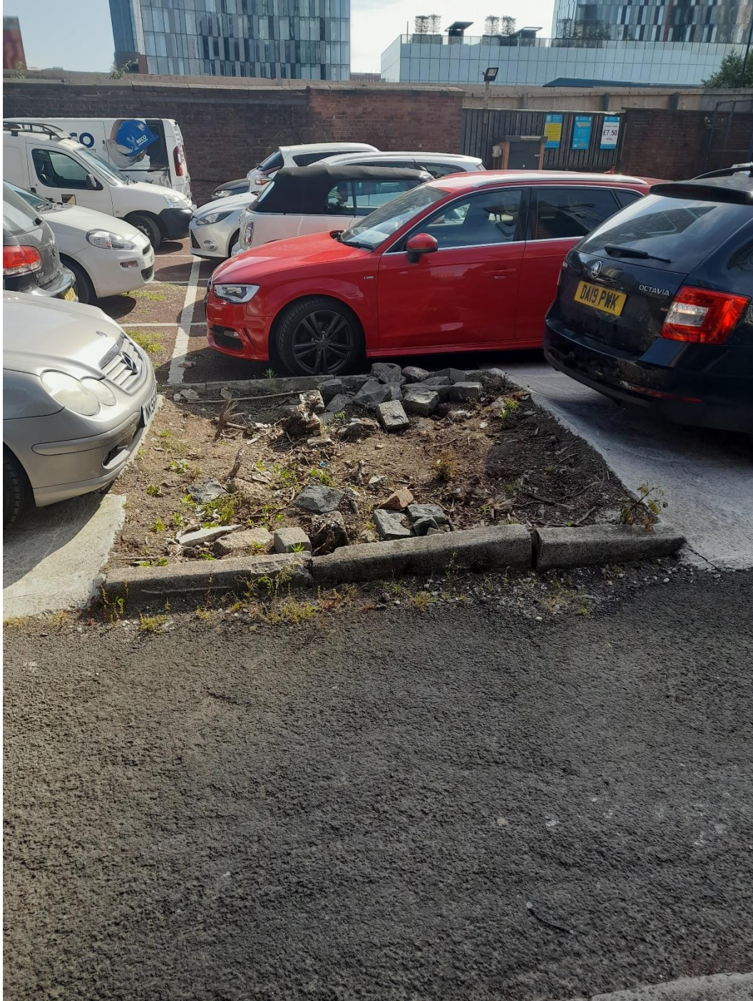
Area of exposed Made Ground noted in centre of car parking area.
