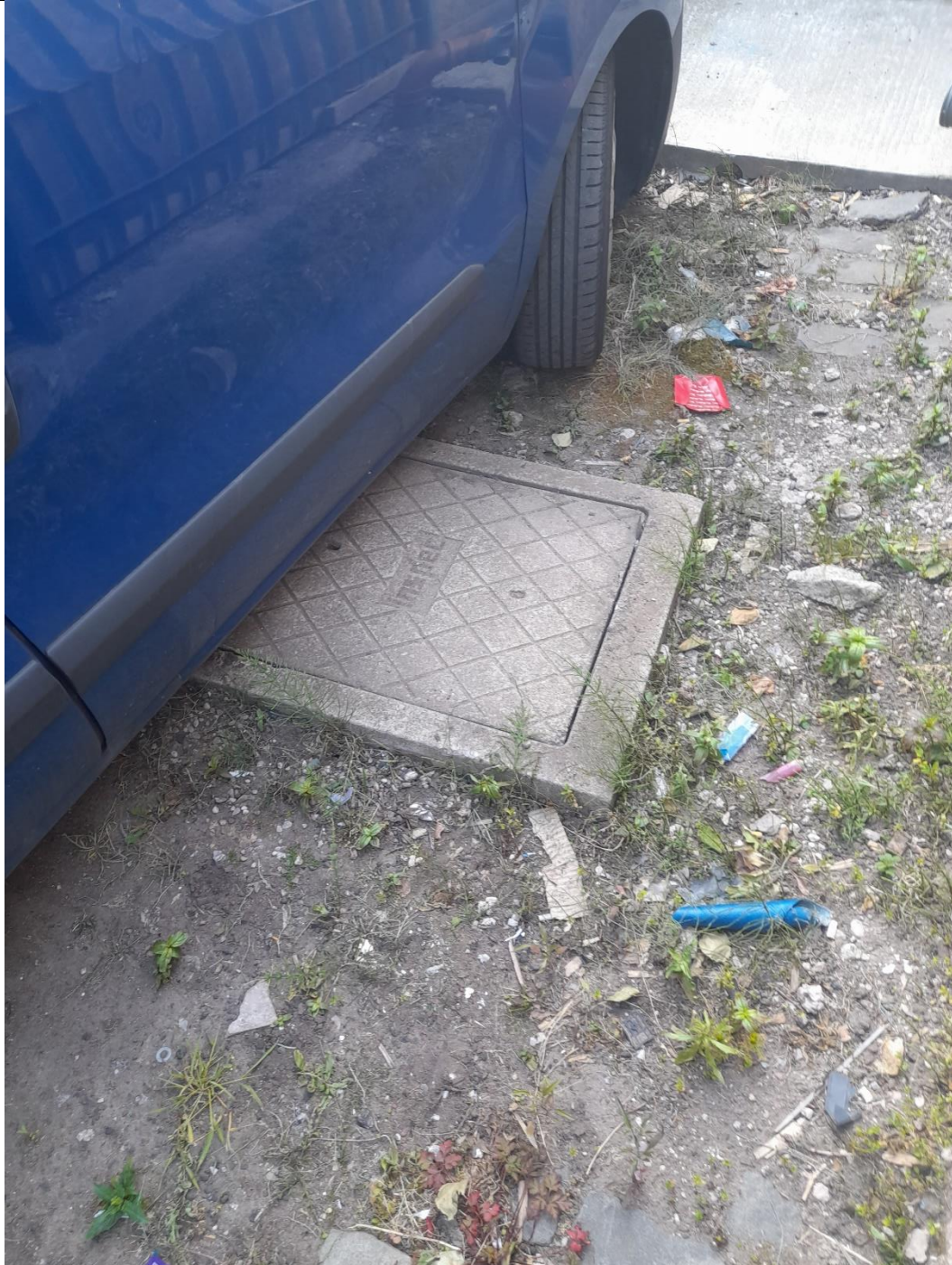
Drainage and service covers noted on the site
