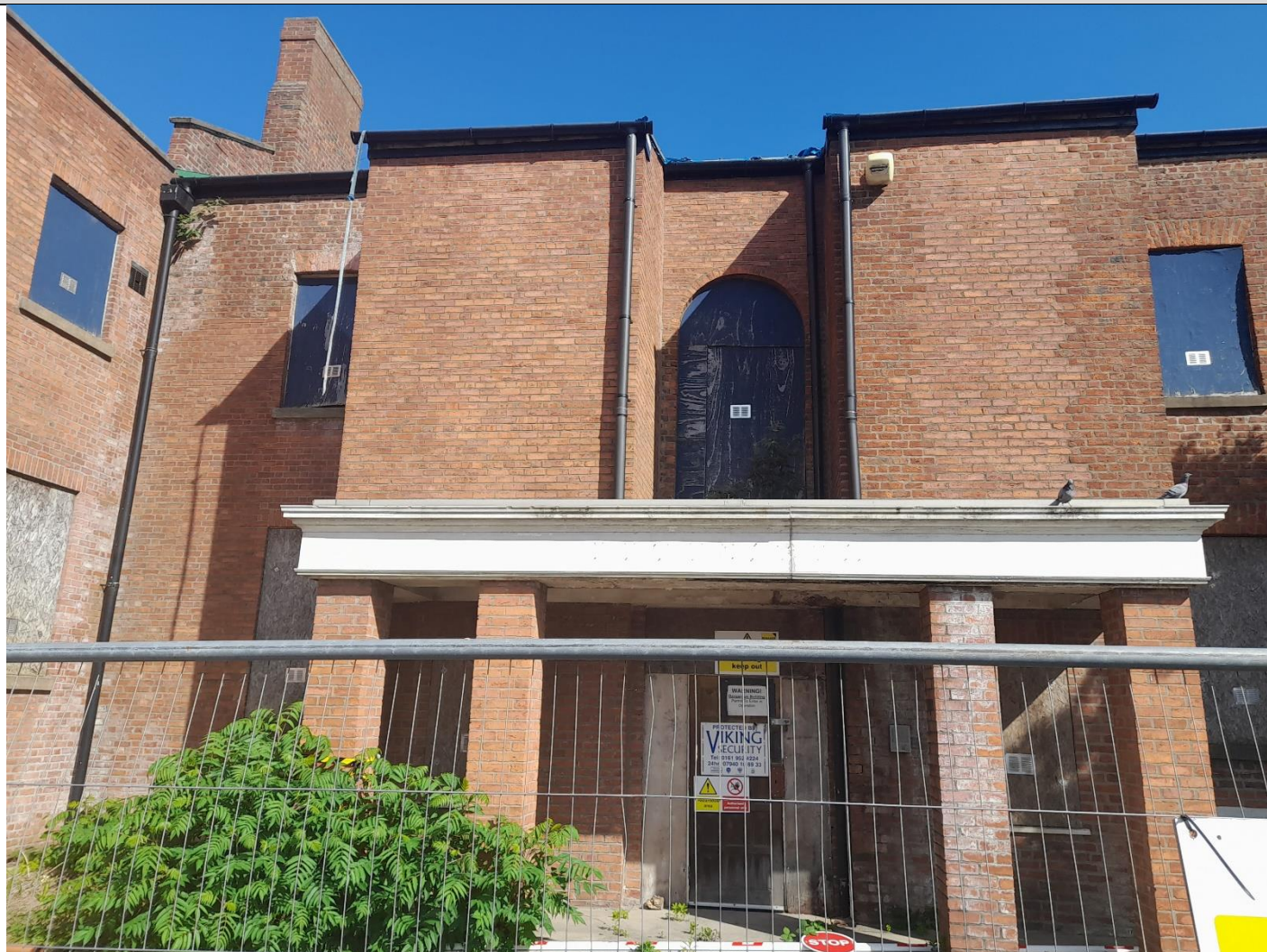
Existing building in northern area of site.
