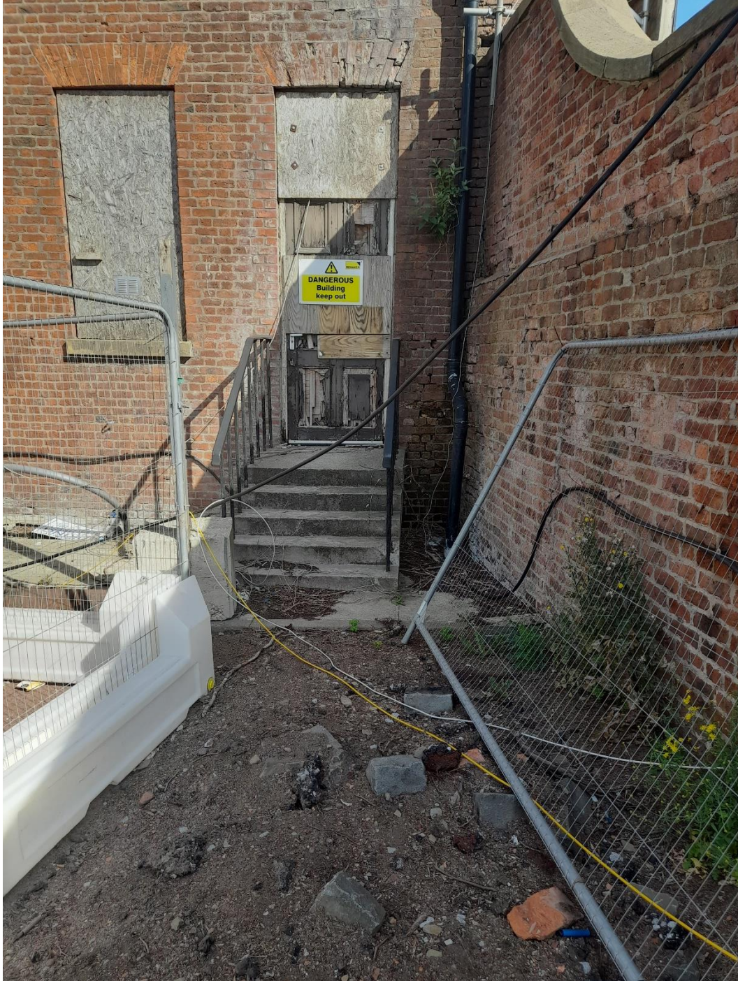
Existing building in northern area of site.
