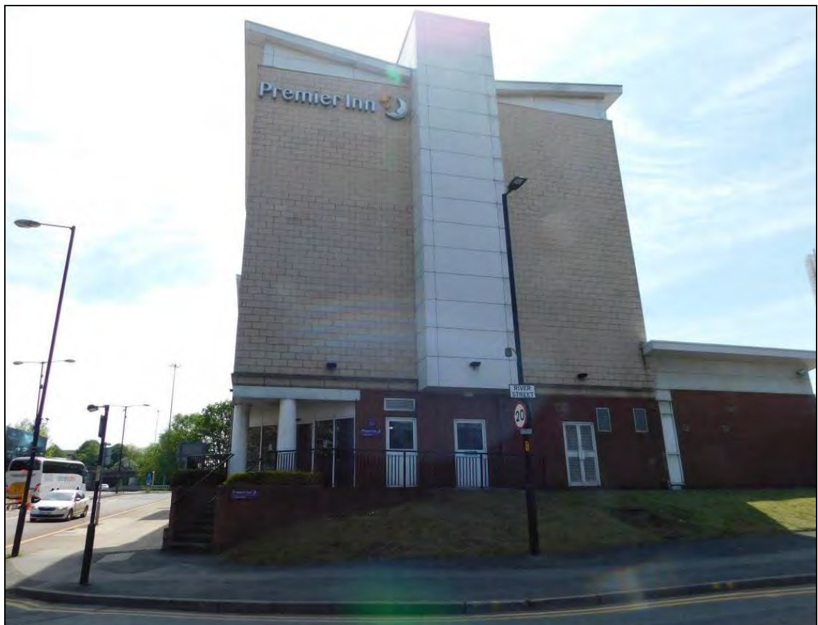
Plate 13: The hotel that occupies the Site at present, the ground floor of which appears to be raised above street level
