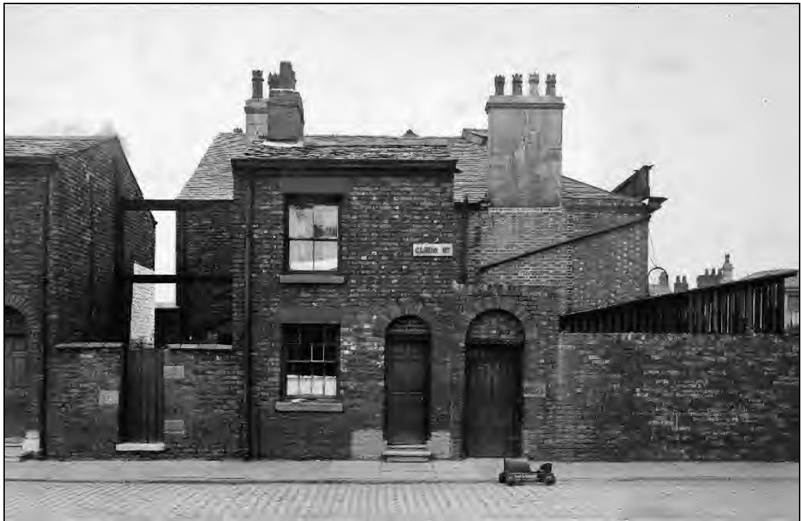
Plate 17: Photograph of Clegg Street house with the Globe Inn to the rear, 1933
