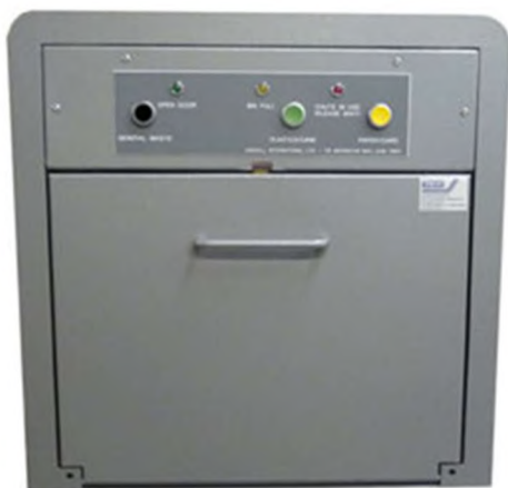
Figure 4.2: Three Way Waste Chute Panel
