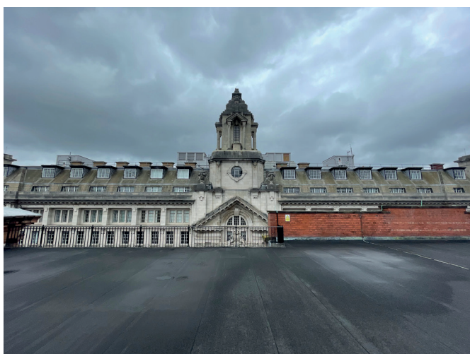
Image 15: Tootal Building roofscape and adjacent St James' Buildings at high level.
