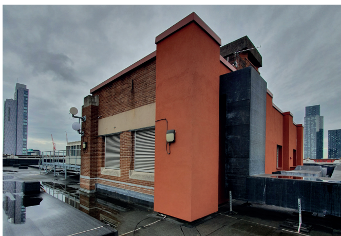
Image 16: Central roof area to Lee House (Rear of Tootal buildings)
