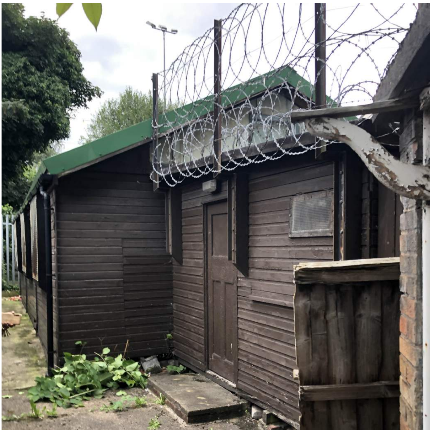
The existing building to be demolished.
