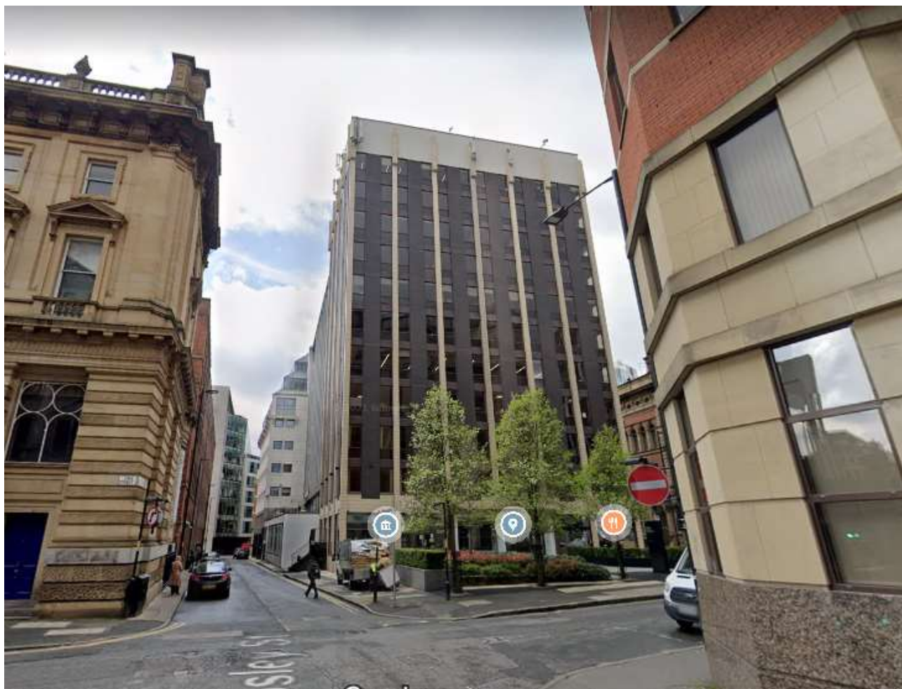
Figure 1: Photo facing York House
