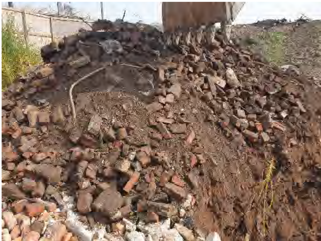
Photo No. 2: TPI01 Arisings
