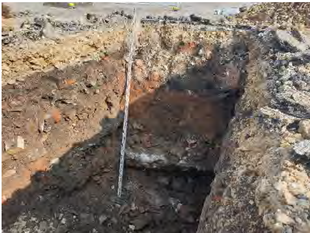
Photo No. 6: TPI03
