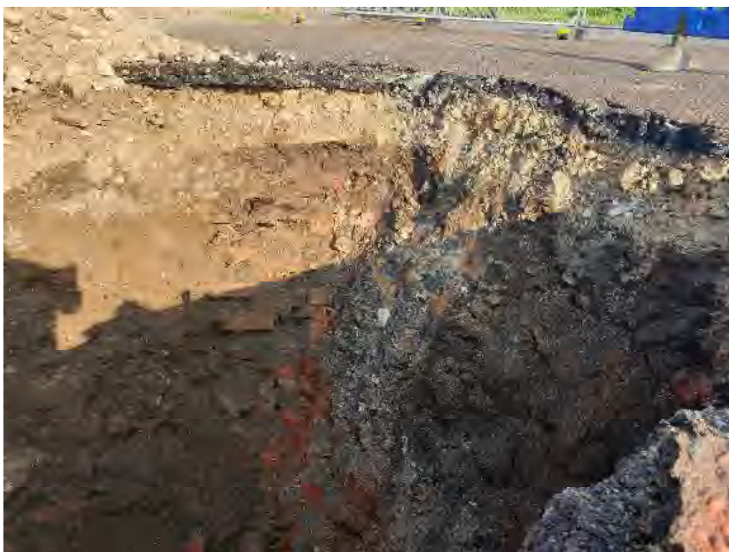
Photo No. 8: TPI04
