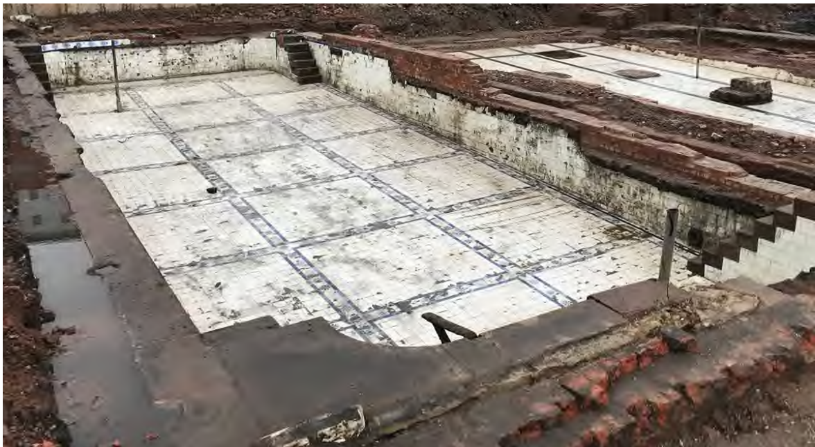
Fig 6.2 : Looking north west across Mayfield Baths former swimming pool.
