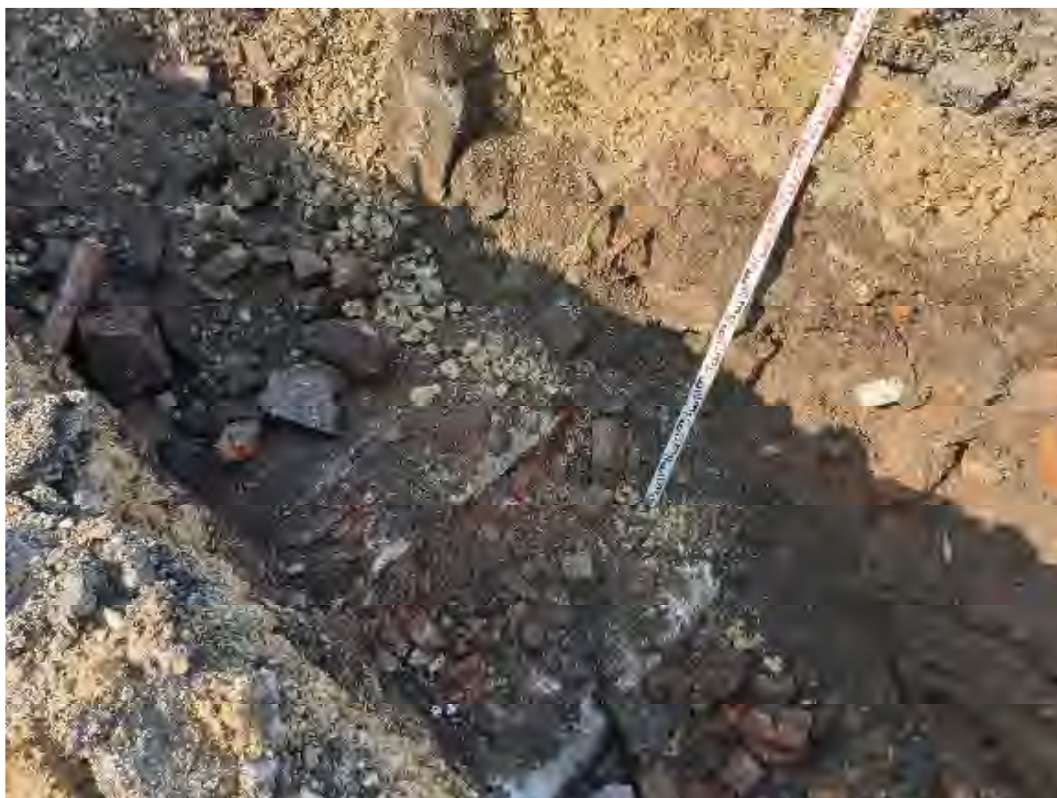
Photo No. 5: TPI03
