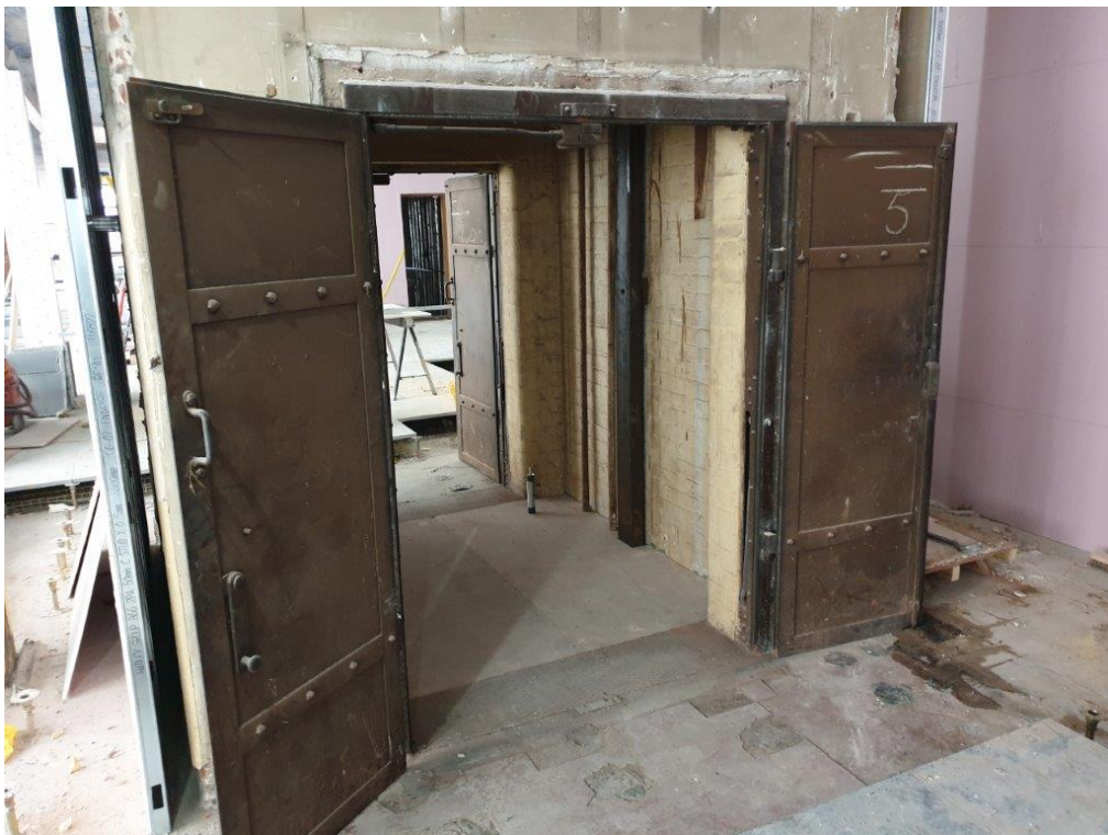
Image 3.3: Revealed historic lift core
