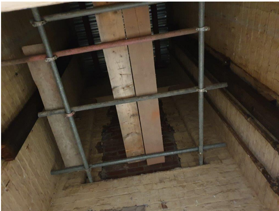
Image 3.4: Revealed historic lift core, from within.
