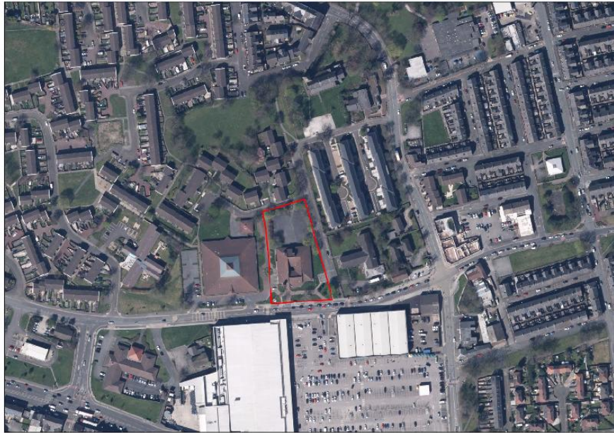
Fig 2 Aerial View of the site
