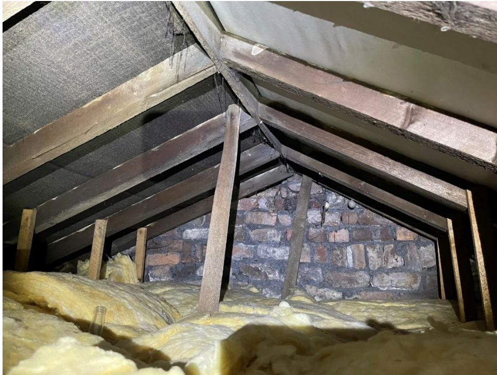
3. Wooden rafters overlain with bituminous felt.
