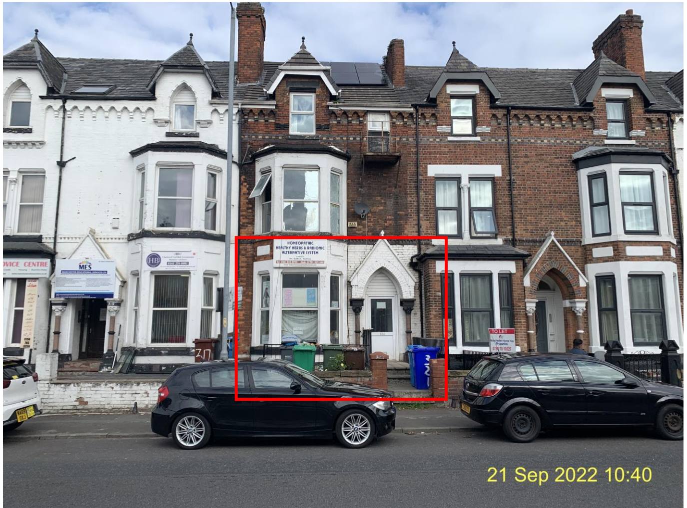
Photograph 1 Site Photograph taken by the case officer
