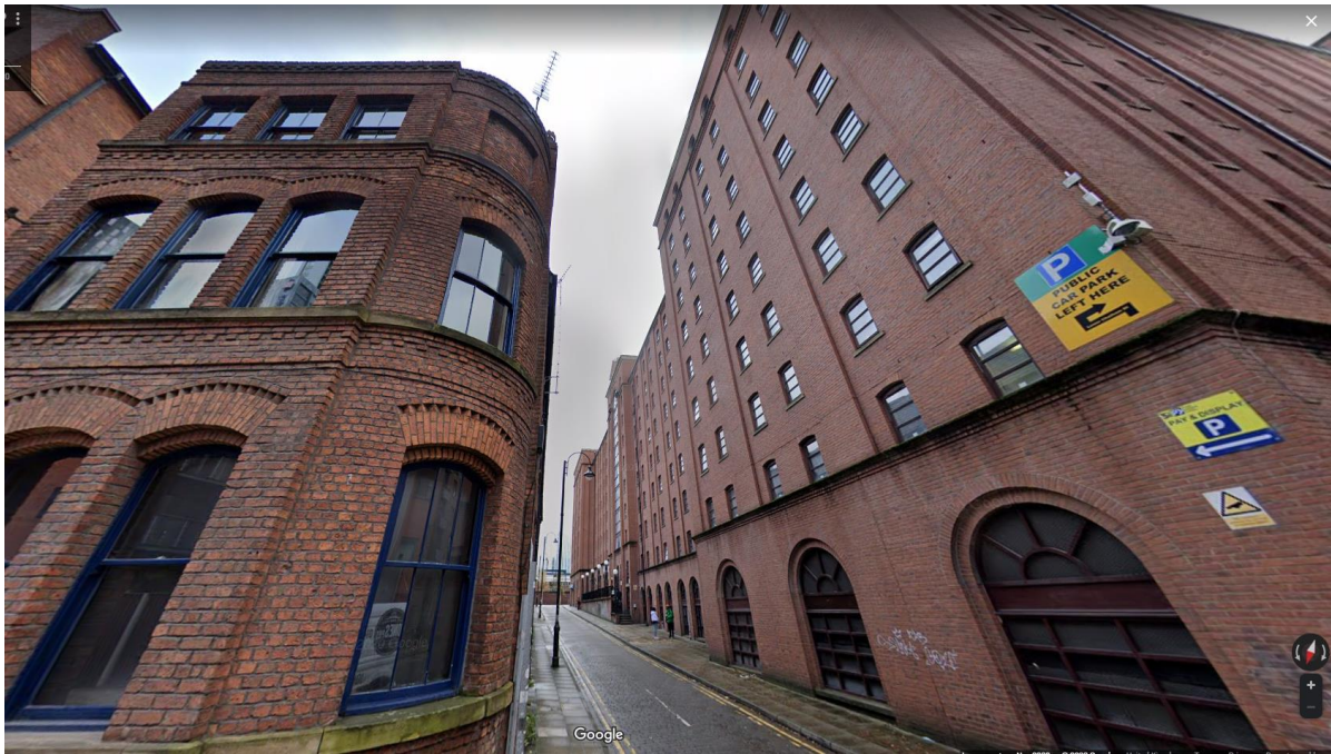
Figure 4. View from north
