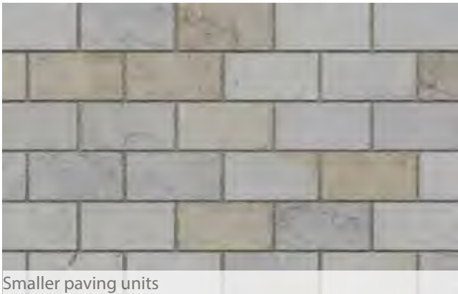
Smaller paving units
