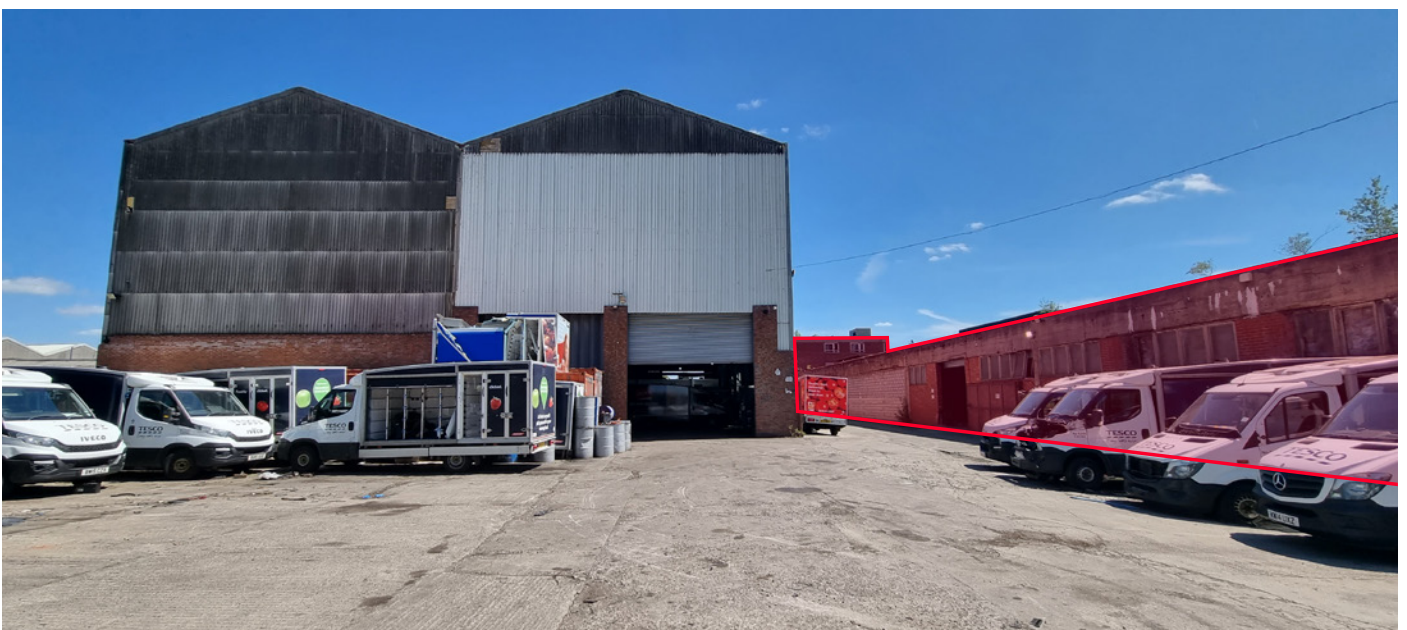
Workshop Building - View B
