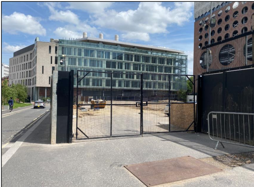
Figure 2.2 – Existing Site Frontage, Viewed from Newman Street Eastbound
