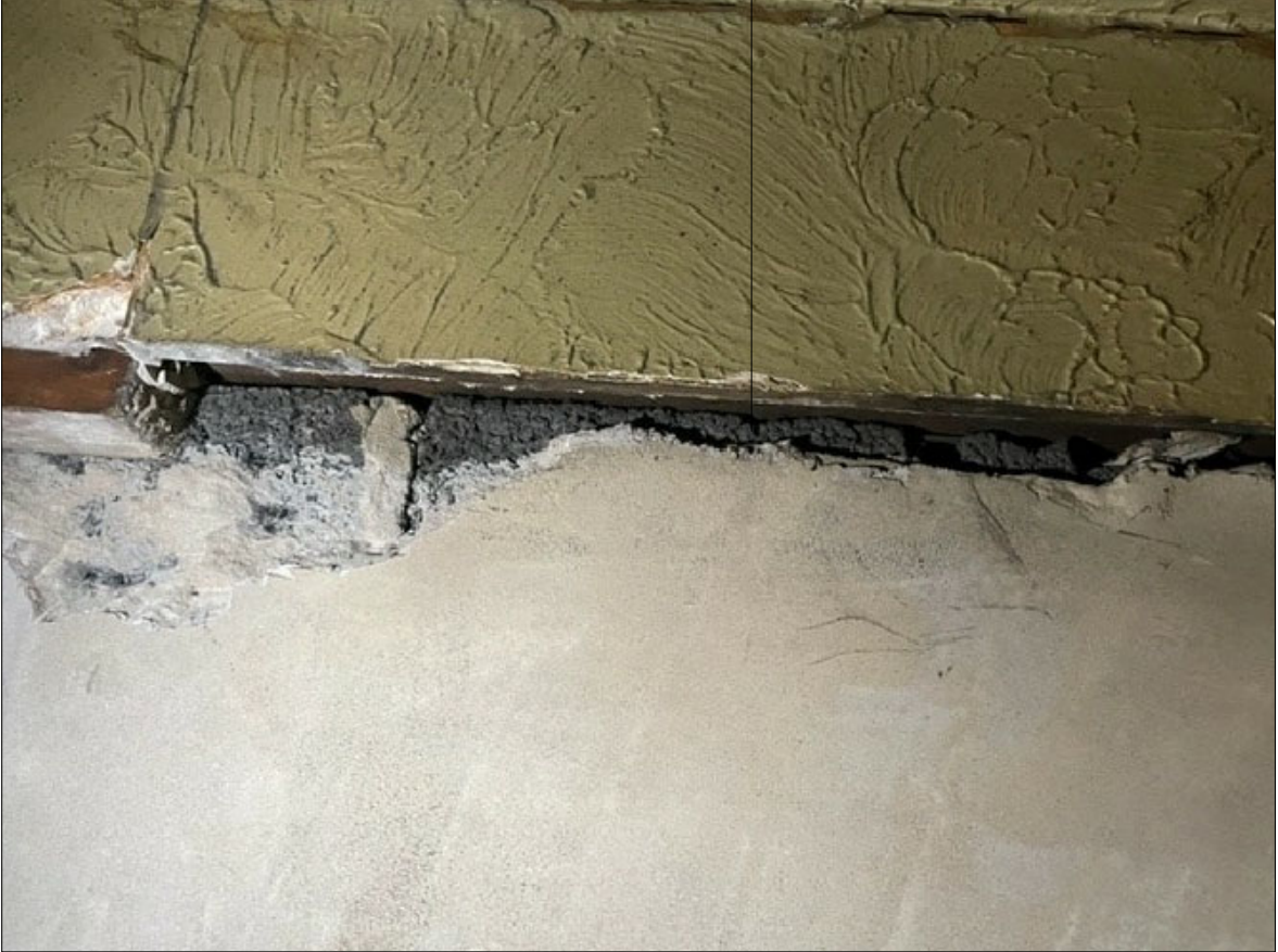
Existing stair enclosure shows modern concrete blocks and therefore not part of the original building
