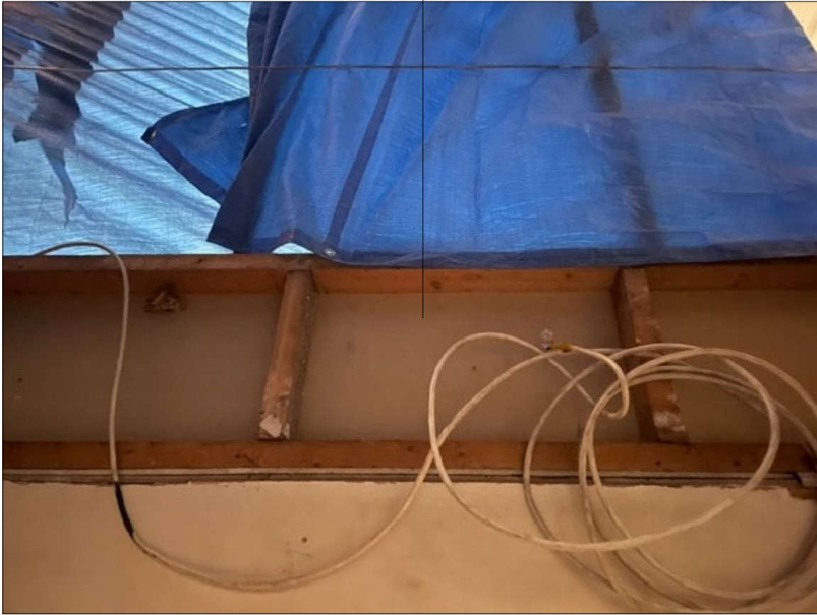
Existing stair enclosure shows modern timber studs and gypsum plasterboard partitioning and therefore not part of the original building
