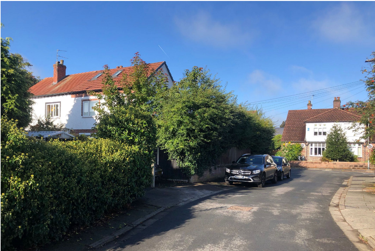
Fig.4: View along Highcroft Avenue towards rear and side elevation with existing garage outbuilding to the left
