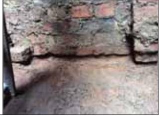
VIADUCT ARCH UNDERSIDE OF FOOTING
